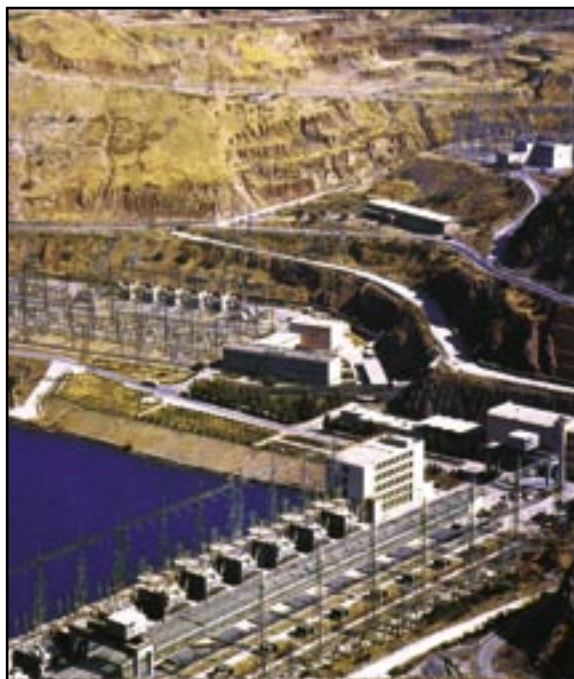
Fig. 21. Nurekskaya HPS, dam height 300 m
