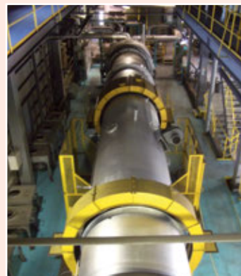
Photo 28: Example of Thermal Treatment (courtesy: Nomura Kohsan Co., Ltd.)
