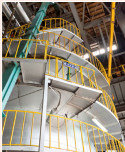
Photo 30: Multiple Hearth Furnace (courtesy: Nomura Kohsan Co., Ltd.)
