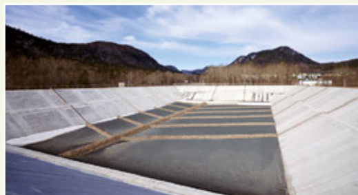
Photo 37: Example (B) of a Specially Engineered Landfill (courtesy: Nomura Kohsan Co., Ltd.)
