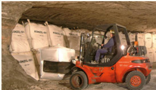
Photo 39: Placement of big bags in the salt mine (courtesy: K+S Entsorgung GmbH)
