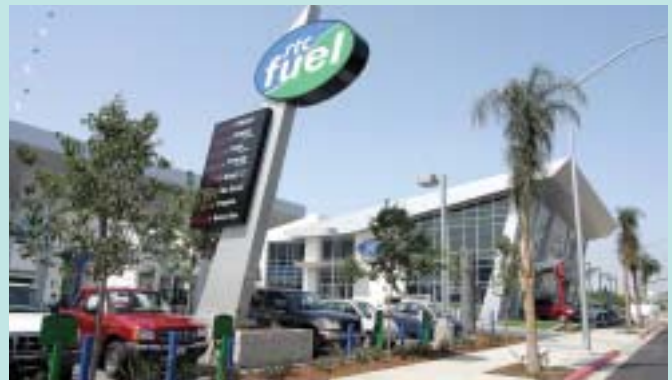
Regional Transportation Center
