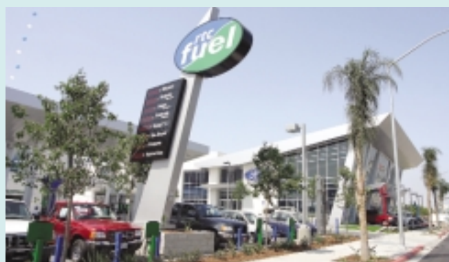
Regional Transportation Center
