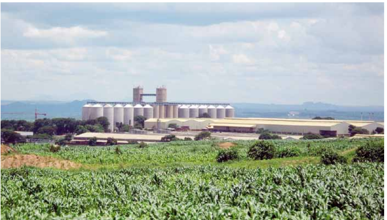
Grain Storage Facility, Photo by Deepa Pullanikattil
