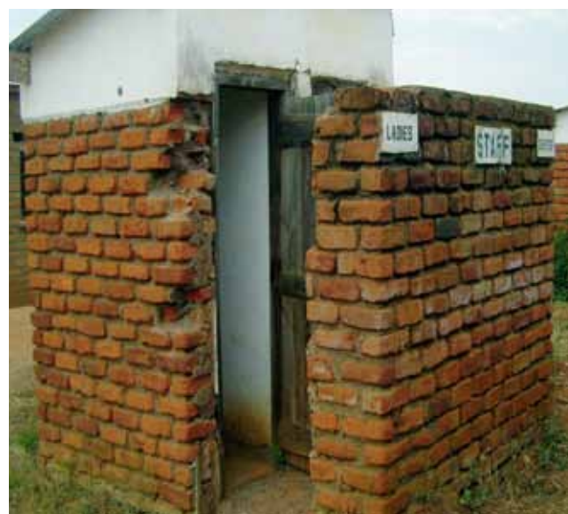
A permanent staff toilet at one secondary school.
