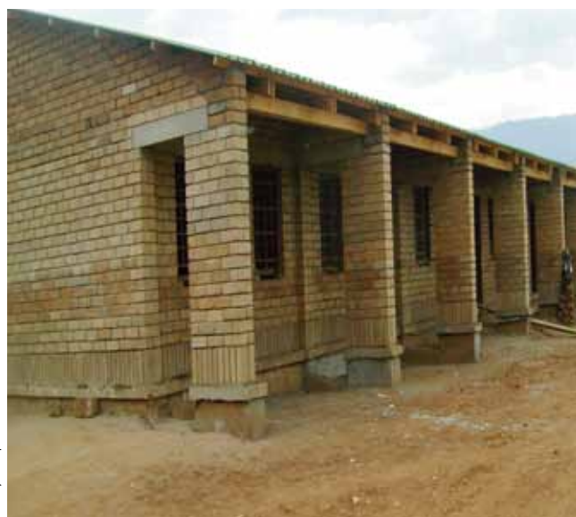
A classroom block constructed with hydra-form bricks.
