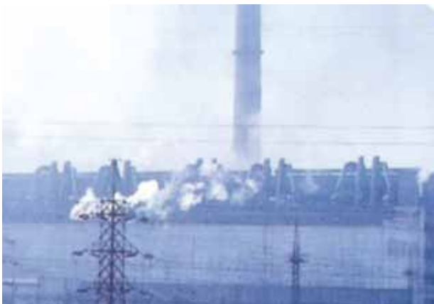
Photo 3.11 Pyongyang thermal power plant
