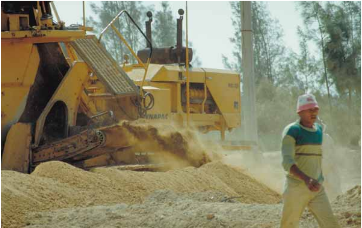
The Egypt-West Beheira underground irrigation system construction site.
