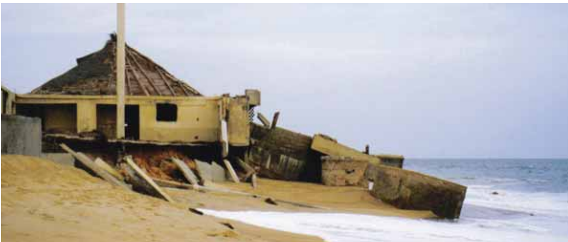
Coastal erosion caused by the interruption of beach sand supply by longshore drift due to nearby port construction at Cotonou, Benin.
