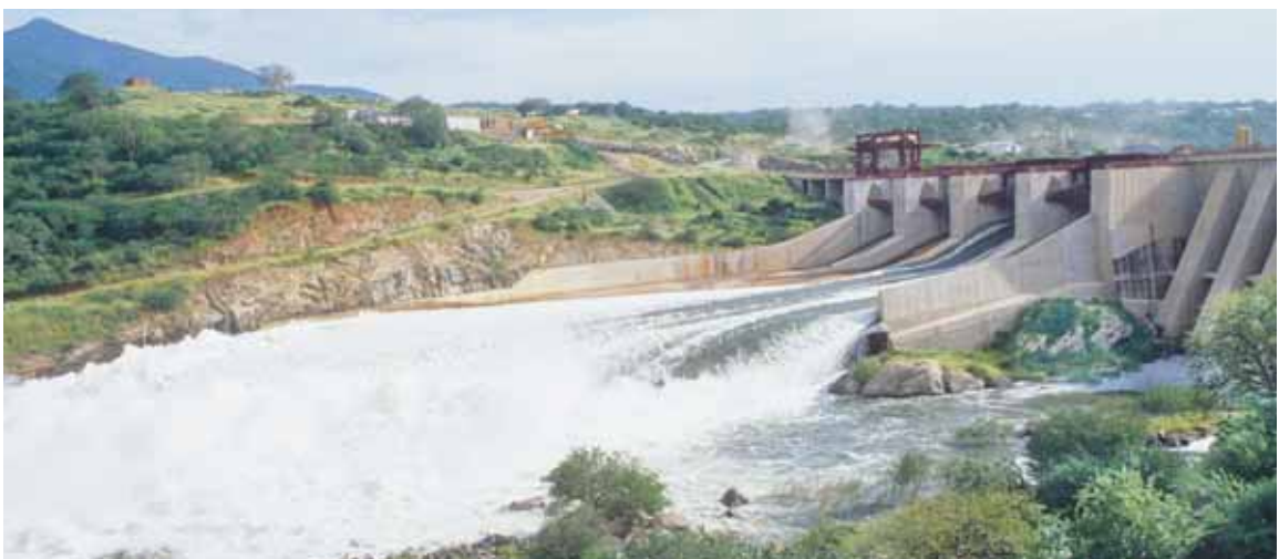
Hydroelectric dam, Tanzania.
