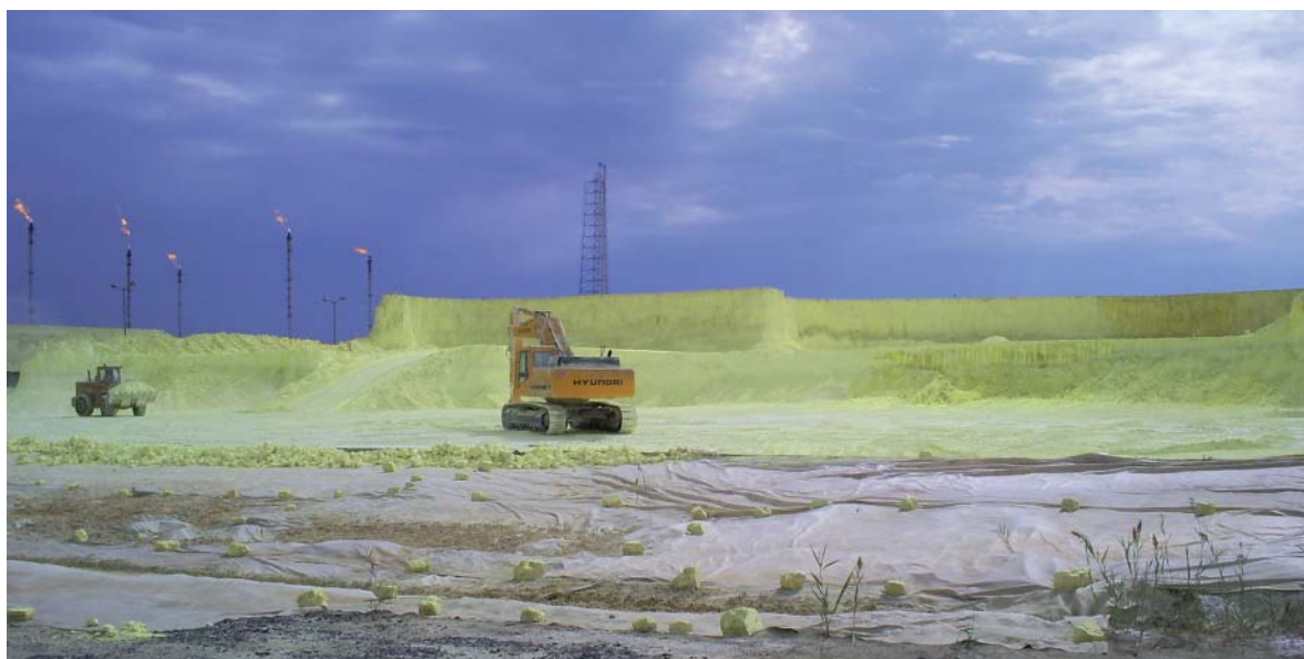
Sulfur pads and flares at Tengiz oil field
