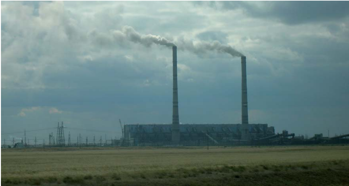
Ekibastuz AES (former GRES-1) power plant
