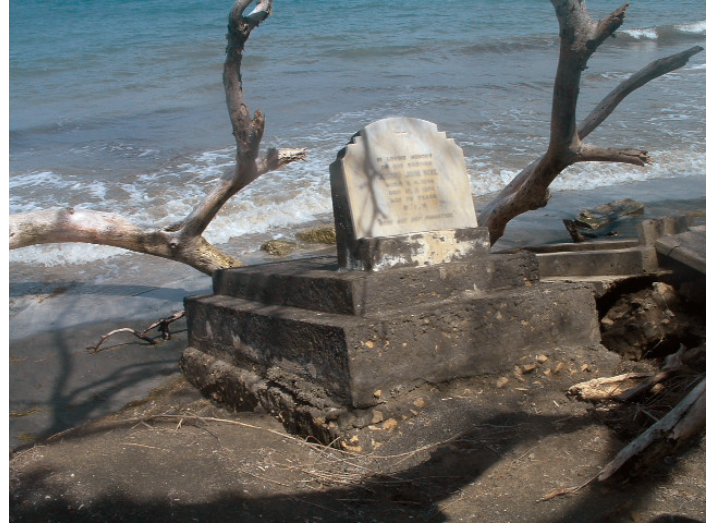
Photo showing beach-side graves exposed by erosion related sand mining. Provided by Suparna Bera, Guyana.
