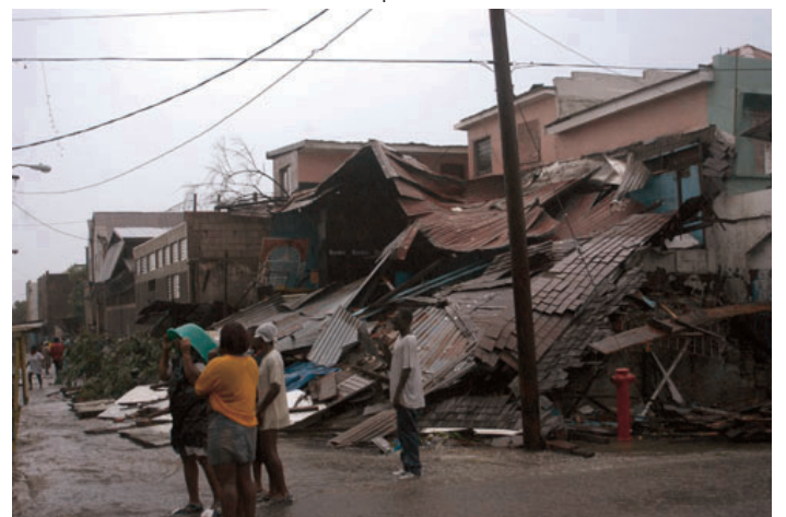
A photo showing a house that has been damaged by the floods caused by Hurricane Ivan, Grenada.
