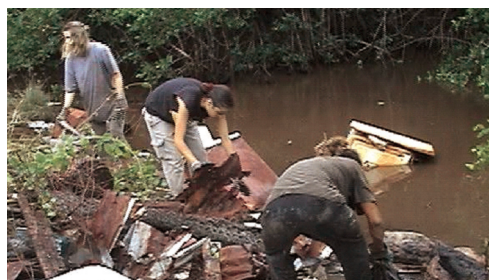
Photo showing the Kilgwyn wetland clean-up project, Tobago. Credits: Environment Tobago, Trinidad and Tobago
