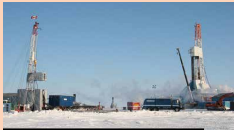
Figure TB-3.2: The Mallik Gas Hydrate Production Research Well, Mackenzie Delta, Northwest Territories, Canada. (Photo courtesy of the Geological Survey of Canada).
