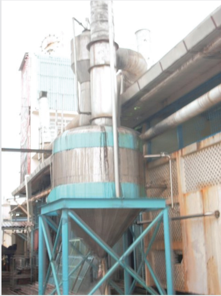
Plate 4.3: Venturi Boiler Emission Scrubber Source: Banks DIH
