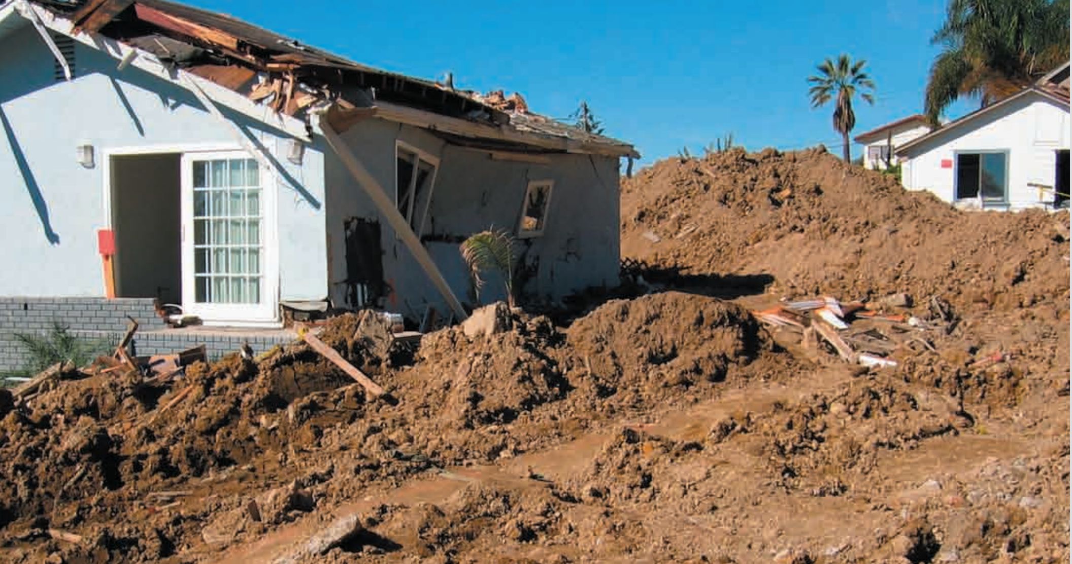
Mudslide Credit: News Photo/UNEP/FEMA
