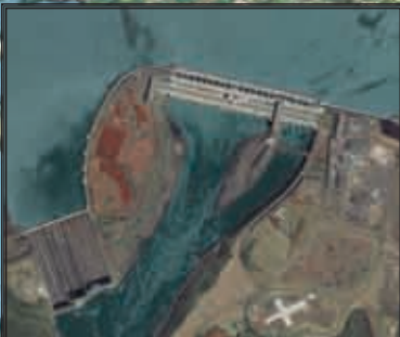
Credit: IKONOS/UNEP/SpaceImaging Itaipú Dam, one of the world's largest, was built from 1973 to 1982 and is a major source of electricity for both Brazil and Paraguay.
