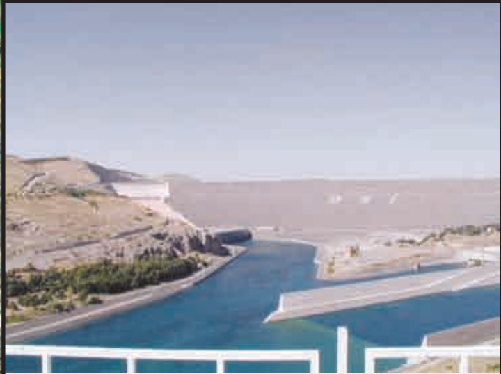
The power-generating station at the Ataturk Dam already provides 8.9 billion kilowatt hours of electricity—roughly 22 per cent of the electricity the country is expected to need by 2010. Credit: Unknown/UNEP/USDA-FAS
