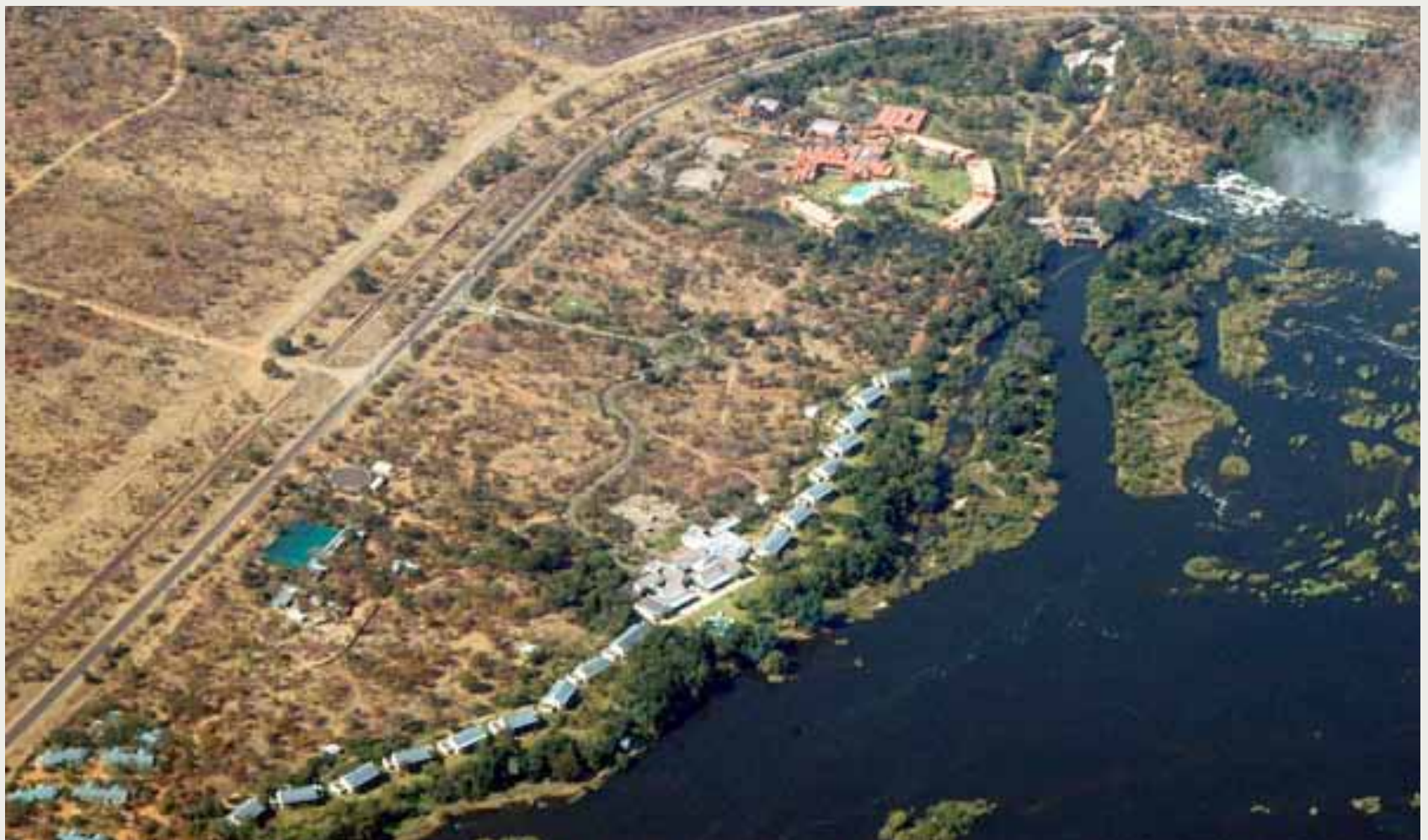
Tourism facilities along the Zambezi River near the Victoria Falls in Livingstone, Southern Province
