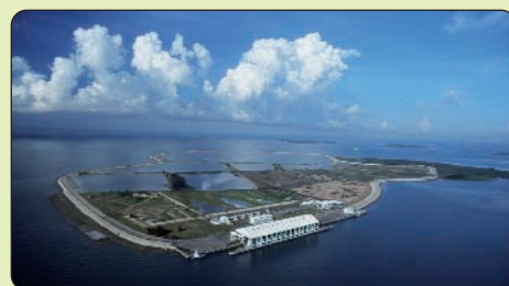
An aerial view of Semakau Landfill
