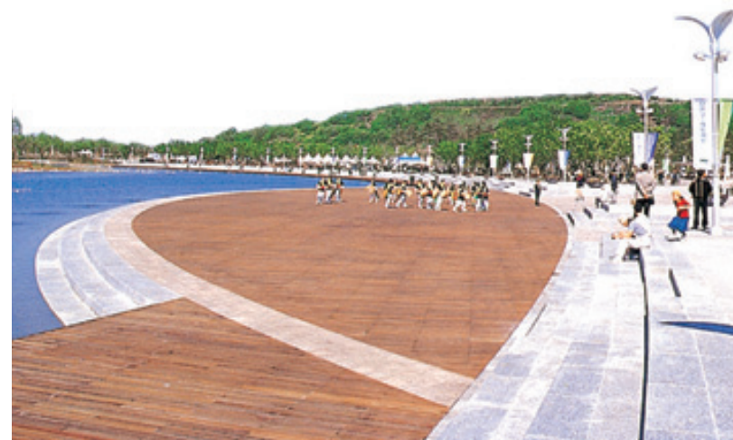
Transformation from a landfill site to a pleasant public space park.
