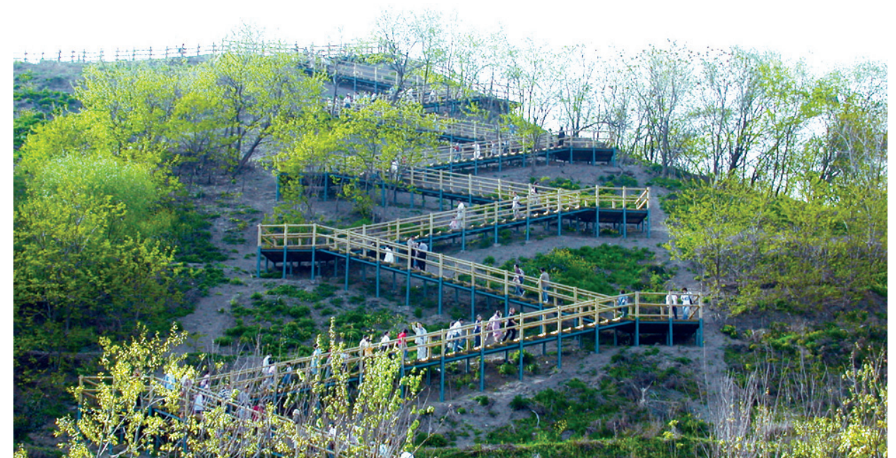
Transformation from a landfill site to the environment-friendly parks.
