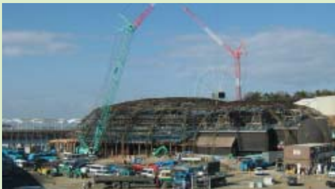
Japanese Pavilion under construction.
