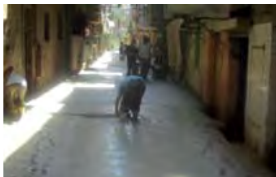
Pic. (9-6) Paving and Constructing Roads
