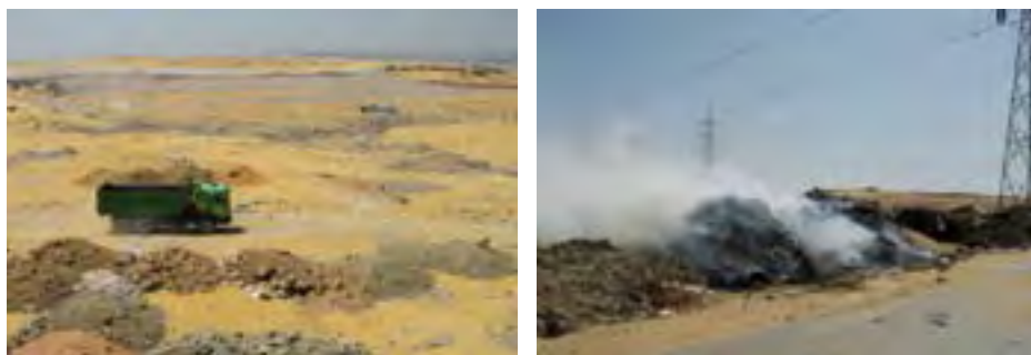
Fig (12-1), (12-2): leveling and covering Al-Wafaa & Al-Amal landfill
