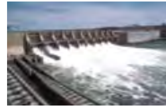
Pic. (5-5) Use of Water in Electricity Generation
