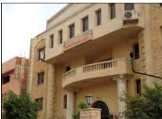
pic (2-4) the monitoring terminal located at El-Mokatam Local Authority building
