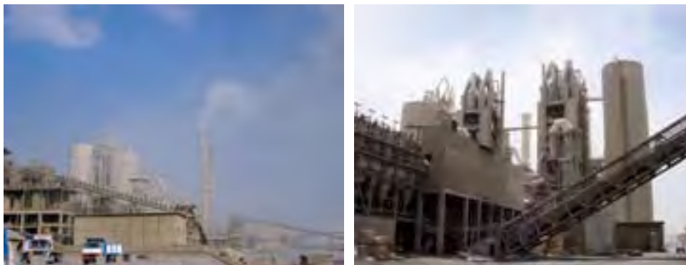
Fig (11-2): Upgrading the old eighth line of electrostatic precipitator.
