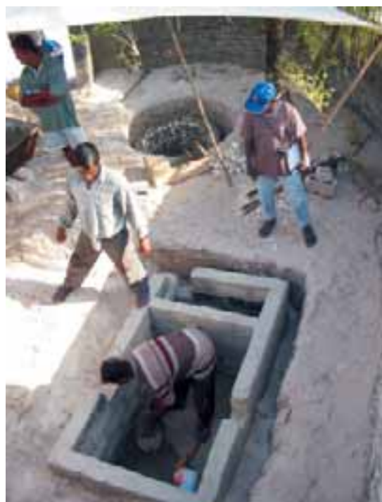
Construction of septic system on HA.Filadhoo Credit: E. Spitaler
