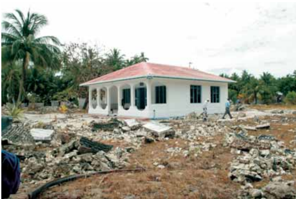
The mosque on K. Guraidhoo survived intact while structures around it were destroyed. Credit: M. Mohammed
