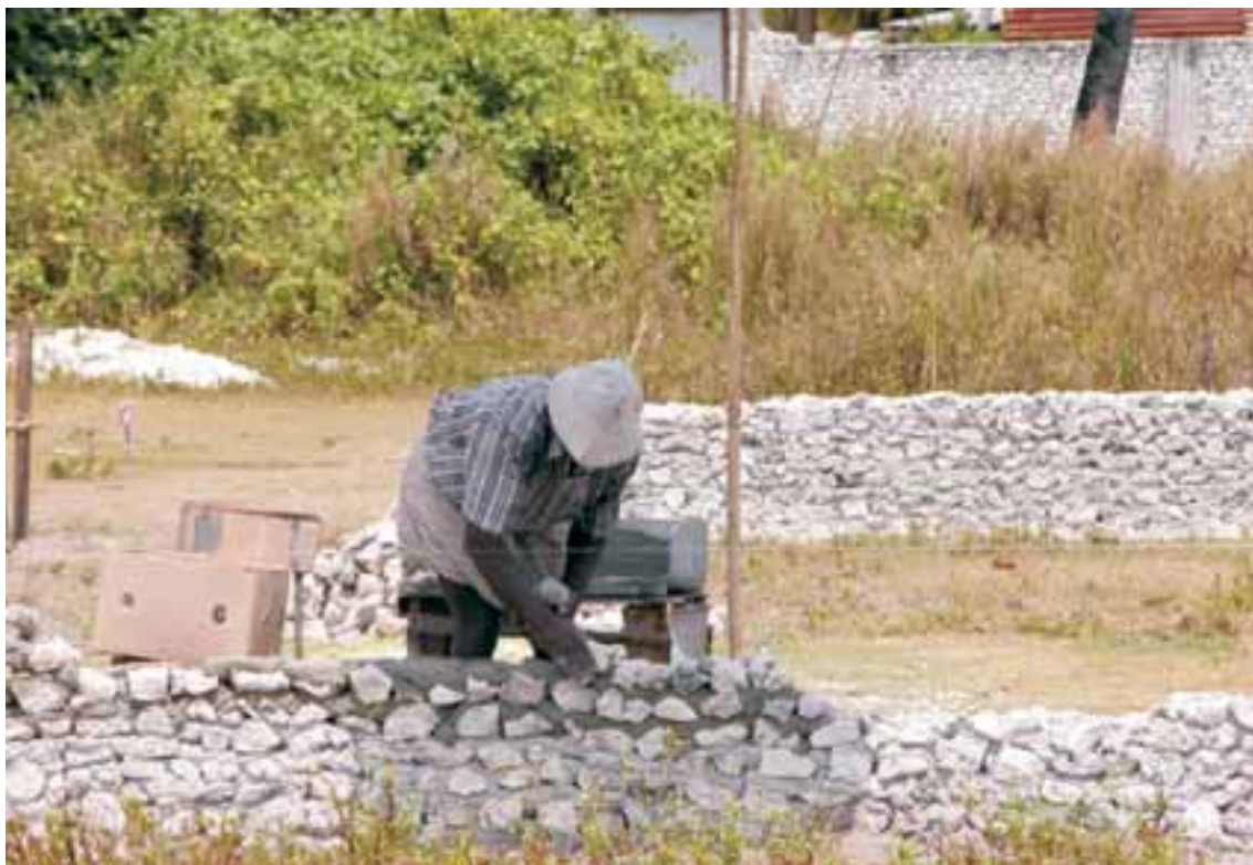
Woman building wall on HD. Kulhudufushi. Credit: J. Bennett
