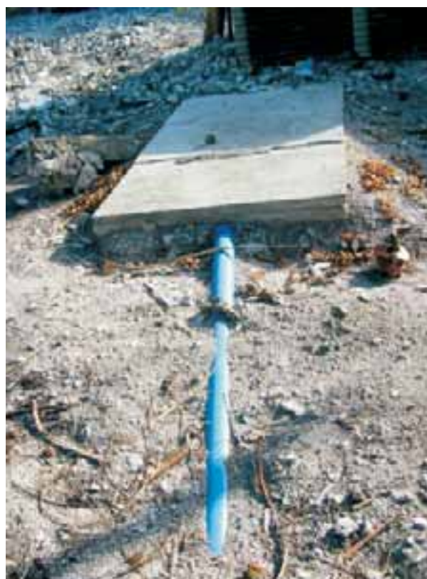
Typical small-scale sedimentation tank on L. Gan. Credit: E. Spitaler
