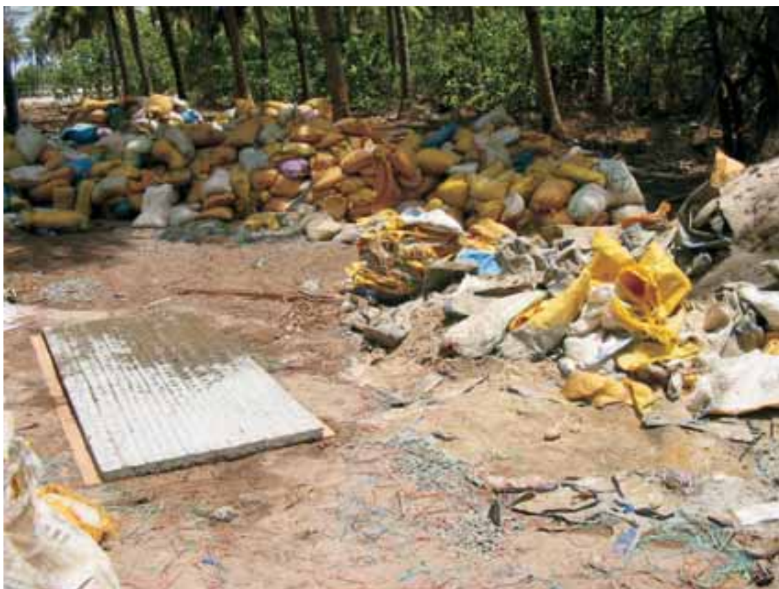
Cement bags and construction waste on K. Guraidhoo. Credit: E. Spitaler
