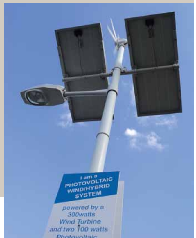
Hybrid street lighting systems in use at the UWI Cave Hill Campus. Photo: Travis Sinckler
