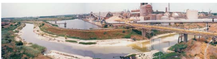
Upper part of Pancevo wastewater canal, 2002
