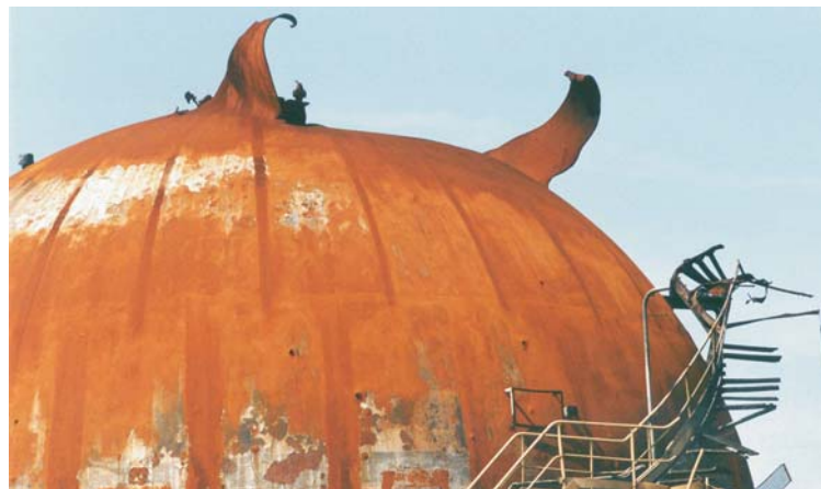
Destroyed VCM storage tank at petrochemical plant
