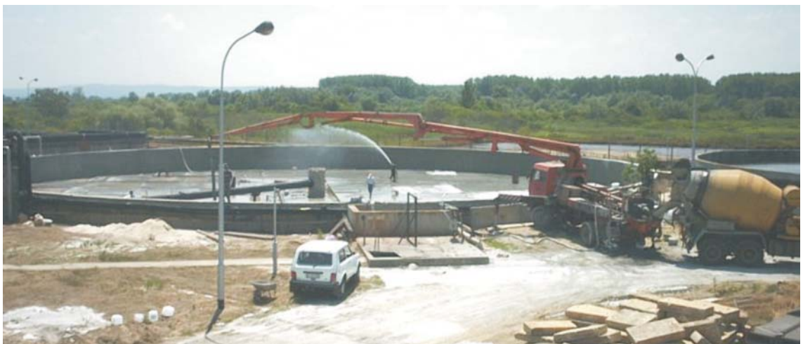
Trickling filter reconstruction
