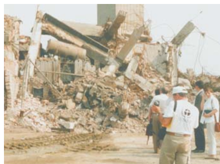
Bor, UNEP assessing contamination risks at transformer station
