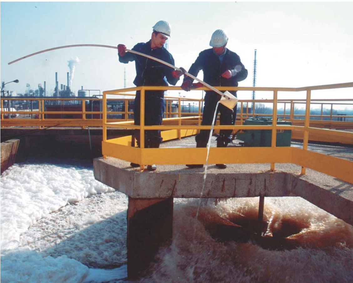
Pancevo petrochemical plant, sampling at wastewater treatment plant
