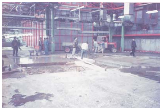
Covering the restored paint hall floor with fresh concrete
