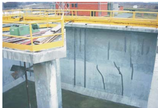
Repaired activated sludge basin interior
