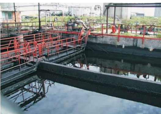
Oil separators prior to rehabilitation
