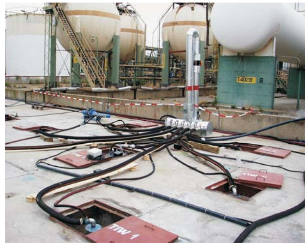
Groundwater remediation, pilot testing
