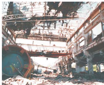
Kragujevac, bomb damage to Zastava factory
