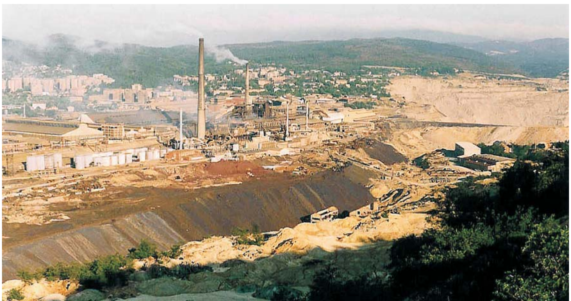
Bor region, the mining complex with the city of Bor visible in the background
