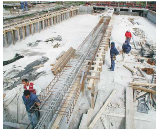
Reconstruction of oil separator's structure at Pancevo oil refinery
