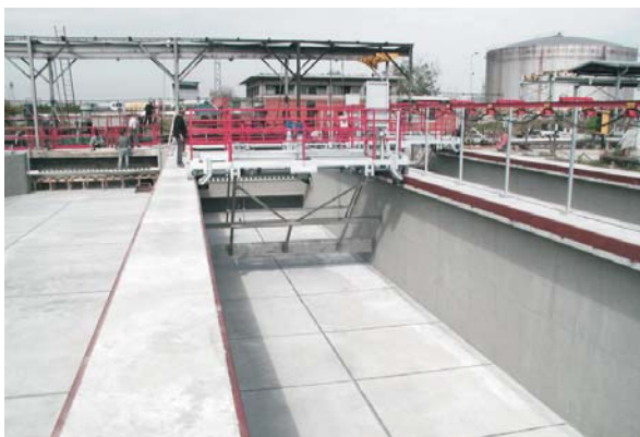
Installation of new equipment
