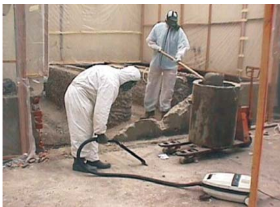
Clean-up works under protective tent at Zastava transformer station
