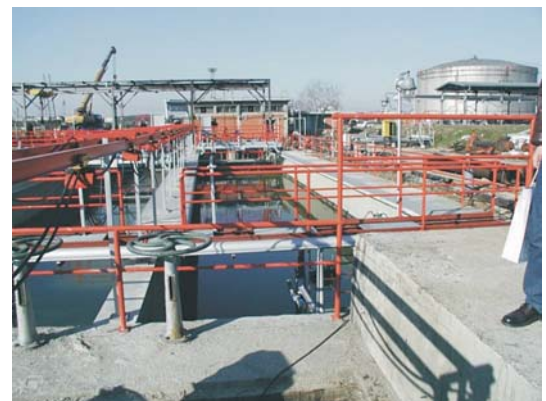
Test run of rehabilitated oil separators
