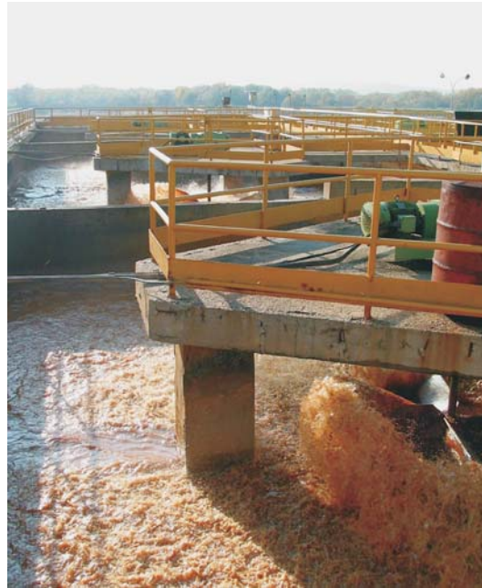
Former activated sludge plant
