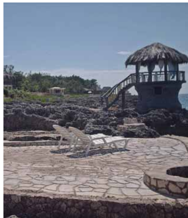
Hotel infrastructure built close to the shoreline and the cliff edge is highly vulnerable to storm surges and wind damage associated with hurricanes
