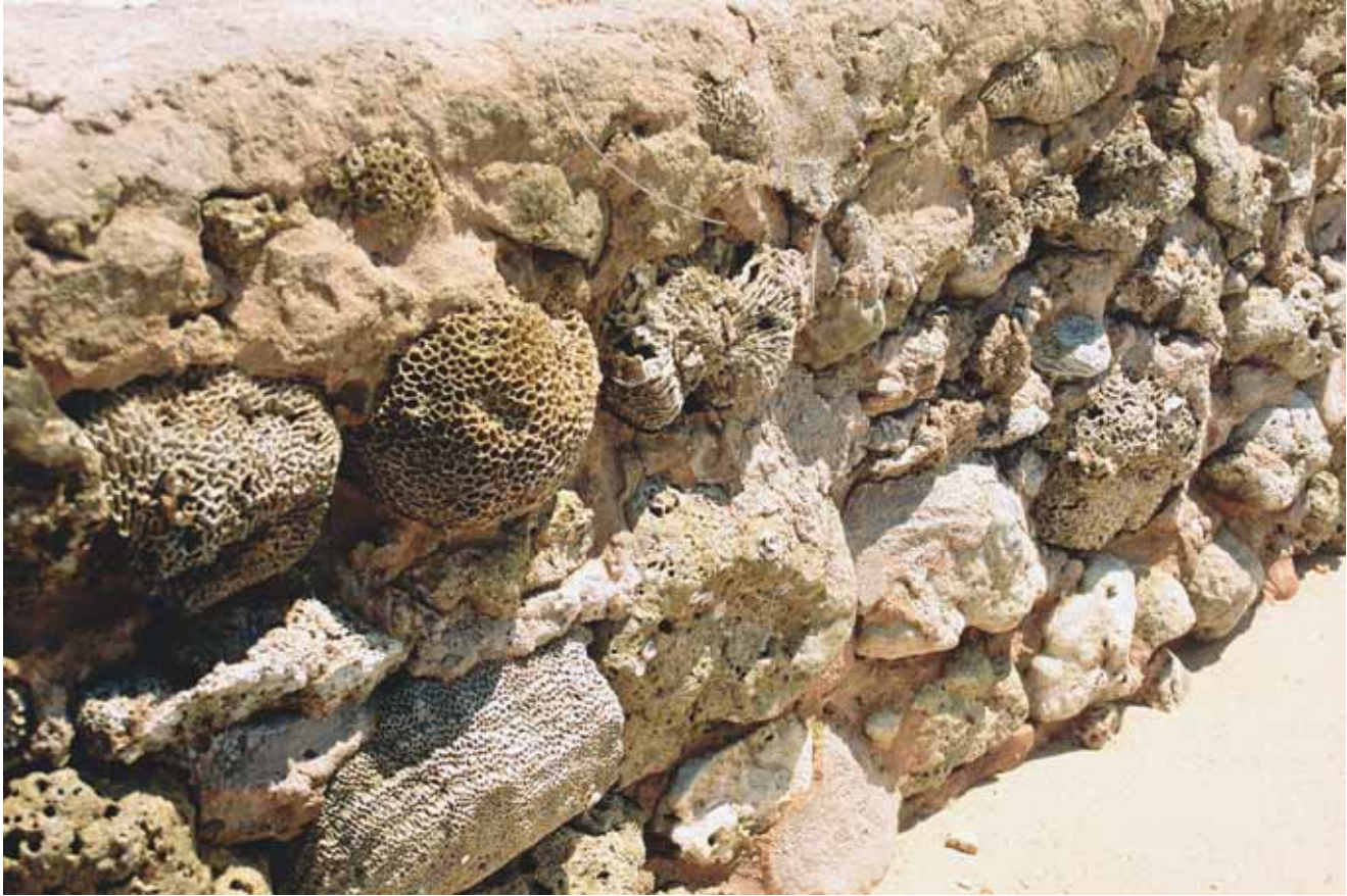
Figure 9 Retaining wall made from coral. (Photo: J. Oliver, Reefbase)
