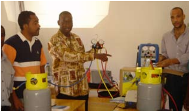
Demonstration on refrigerant recovery in Cape Verde
