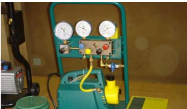
Final step of hydrocarbon retrofitting
