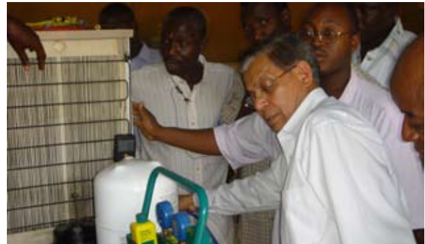
Retrofitting of a R-12 refrigerator to hydrocarbon in Burkina Faso
