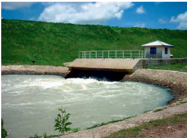
Figure 36 The Tiga Dam (Hadejia river system, north Nigeria). (Photo: Oguntola 2003)
