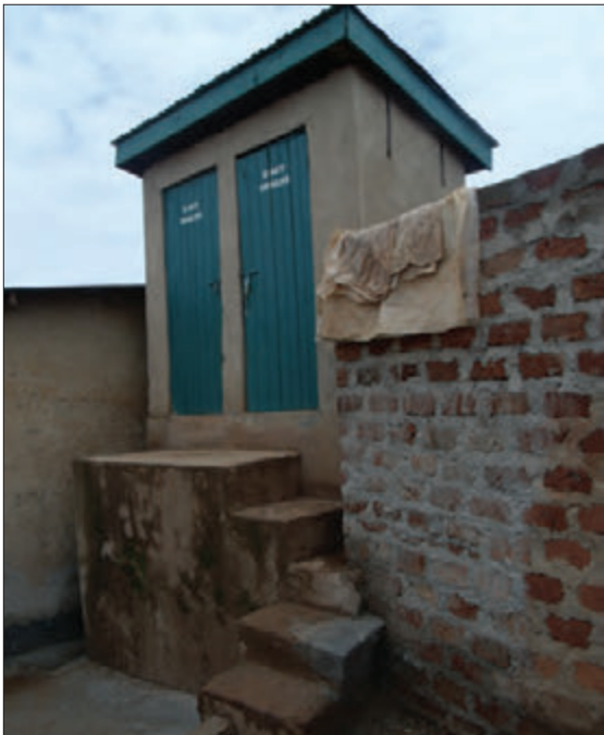
A raised pit toilet
