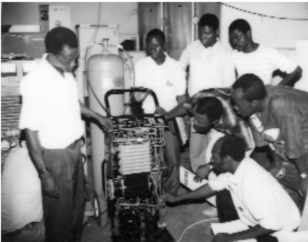
Refrigerant recovery and recycling demonstration in Ghana. Training and certification of servicing technicians are a key to ensuring a successful RMP.
