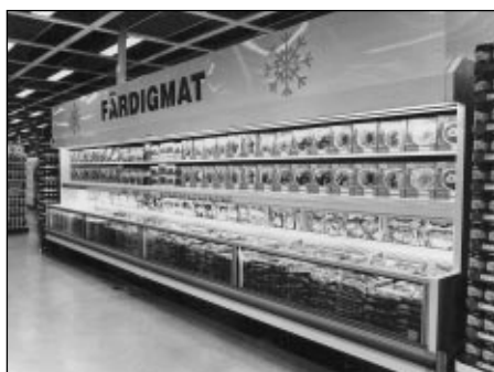
One of the coolers in the 3000 m 2 AGs Favor supermarket in Helsingborg, Sweden, now dependent on hydrocarbon refrigerants.
