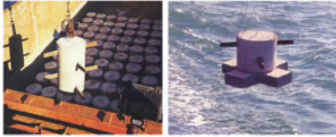
Fig 2.3. – Concrete structures with deterrent elements (General Secretariat of the Sea, Spain).
