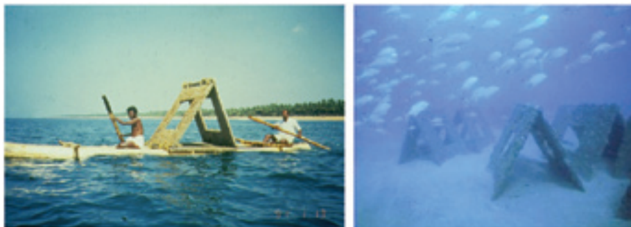
Fig. 1.4.9. – Ferroconcrete artisanal fishery reef units, Kerala, southern India (Source: left: Alternative Technology; right: Antony Jensen, NOC).
