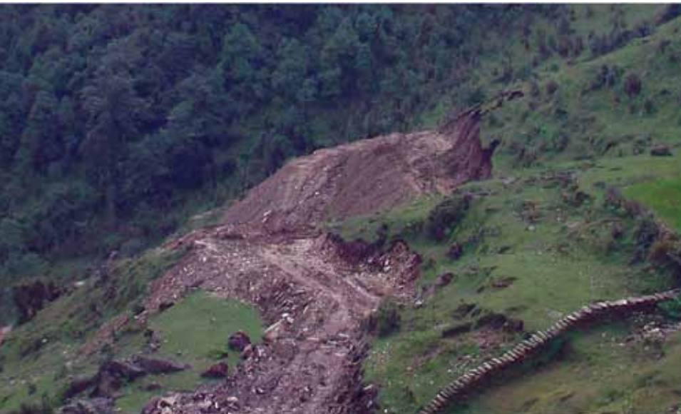
Landslide events like this one are common on Village Development Committee roads (PEI Nepal).
