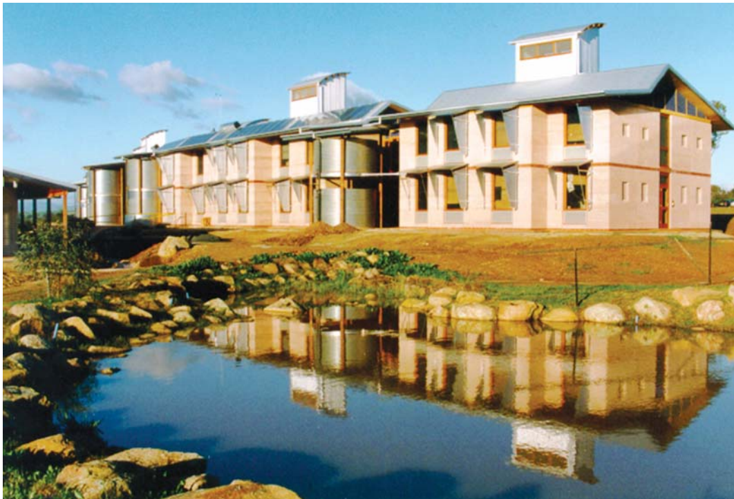
Figure 4: Thurgoona Campus - CHARLES STUART UNIVERSITY, NEW SOUTH WALES, AUSTRALIA. This Campus building incorporates sustainable construction, bio-climatic and water-sensitive design in an integrated "learnscape" - a physical example of and setting for education in sustainable development.
