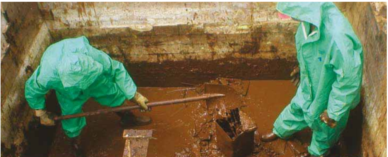
Removal of contaminated sludge from electroplating tanks in Al-Qadissiya. Credit: UNEP/Post Conflict Branch 2006
