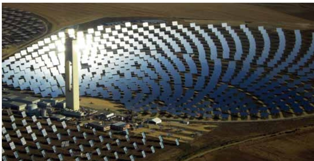
In Spain, new solar panel plant PS20 is under construction next to plant PS10. At a height of 115 metres, PS10 is powered by 624 mirrored heliostats. At 165 metres, PS20 is powered by 1 255 of them. PS20 has been designed to produce twice the energy of its smaller, 11 MW neighbour. Although not the world's first 'power towers', these are the first such plants conceived on such a scale.
