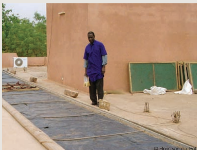
Present director of USISS with the double solar tunnel dryer (drying racks against the wall of the handling room). Source: USISS
