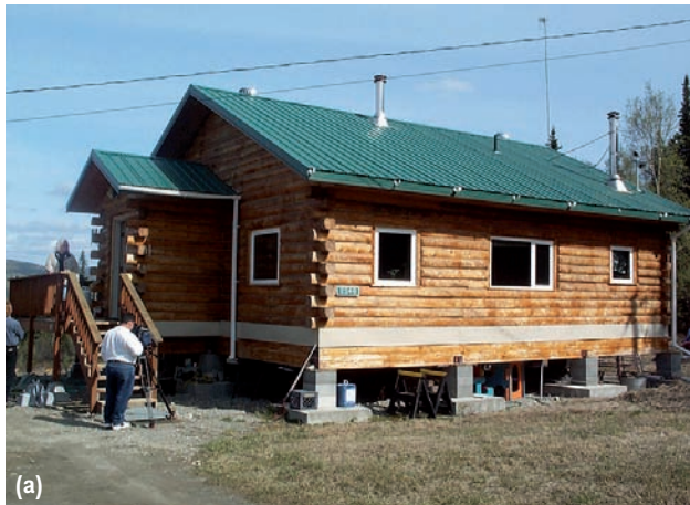
Figure 7.7: Examples of good engineering practices which prevent permafrost thawing.
