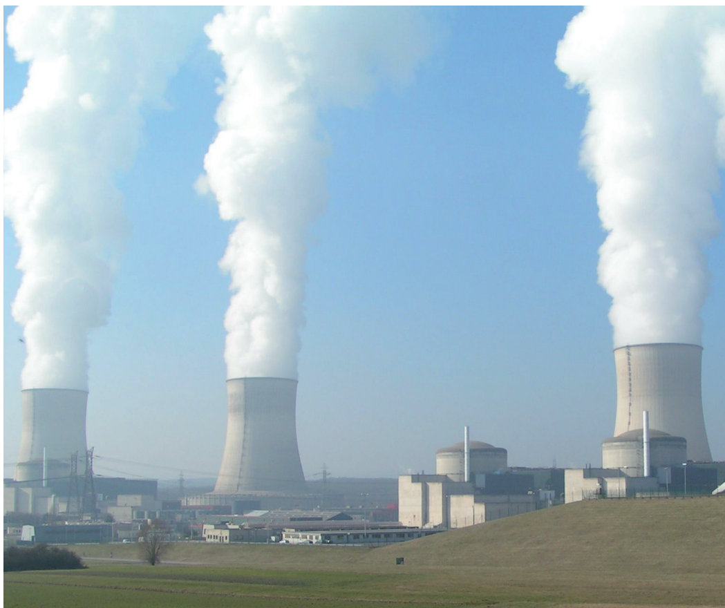
The nuclear power complex at Tricastin in southeastern France
