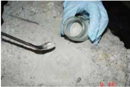
Picture 19: Sampling of concrete
