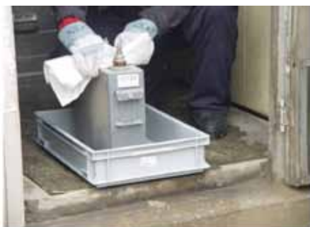
Picture 67: Phase out and cleaning of PCB capacitor
