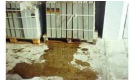
Picture 85: Bad example II (no tip trays)
