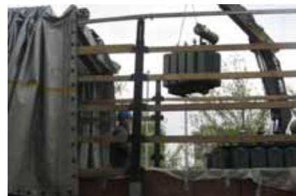
Picture 71: Loading of transformers
