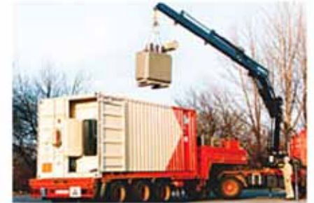
Picture 100: Loading of transformers
