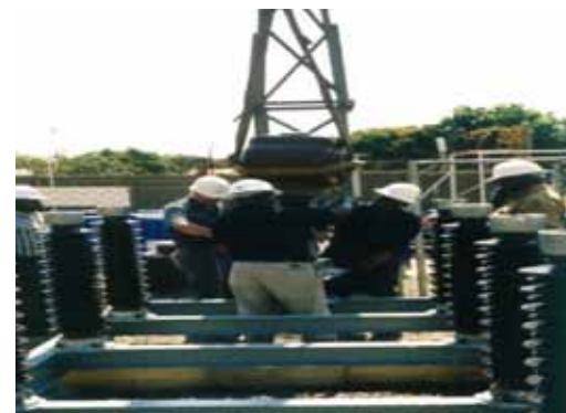
Picture 55: Dismantling of capacitor battery
