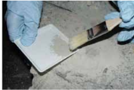
Picture 20: Cleaning of leftover dust
