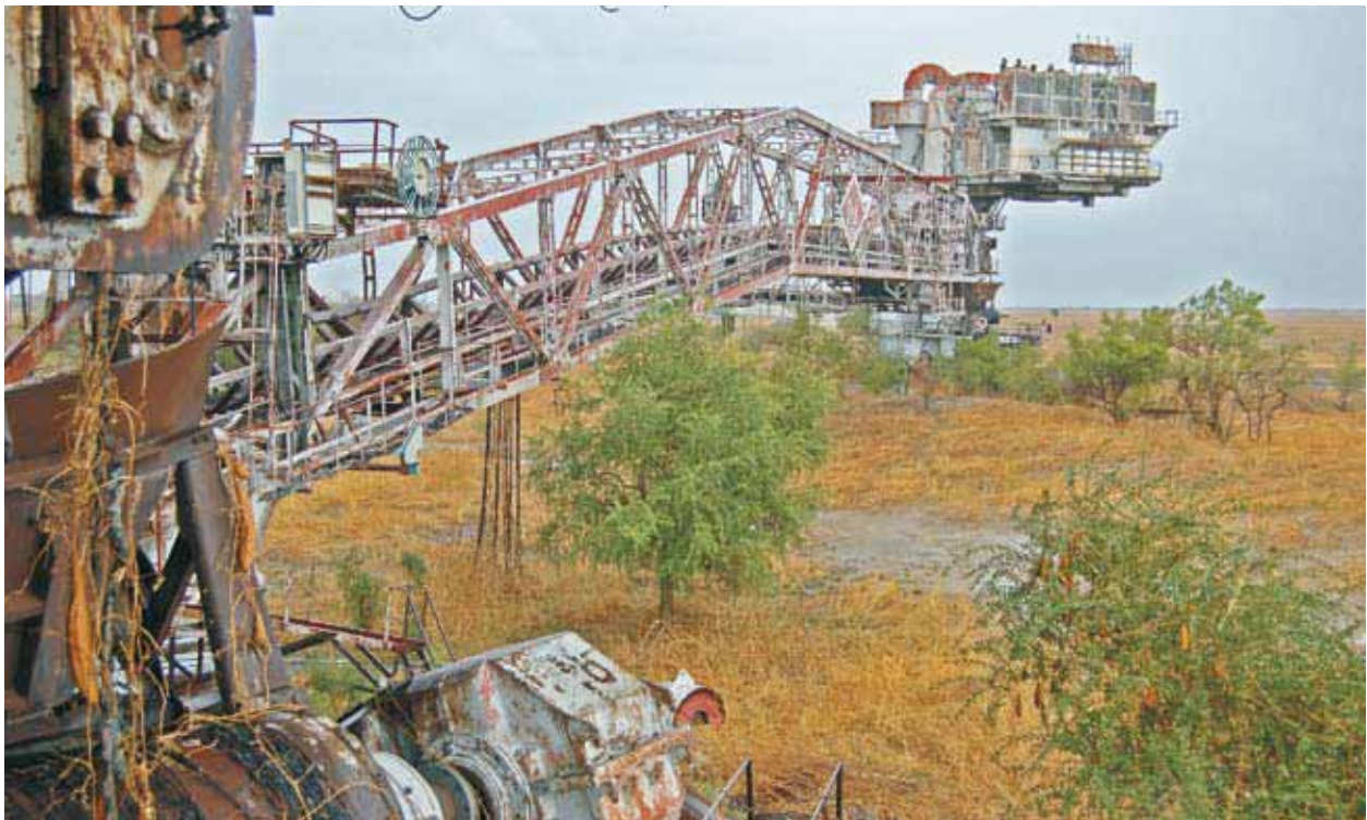
The main excavator for the Jonglei canal is composed of several self-propelled sections. Once the largest of its type in the world, it now lies in a derelict state in the canal bed
