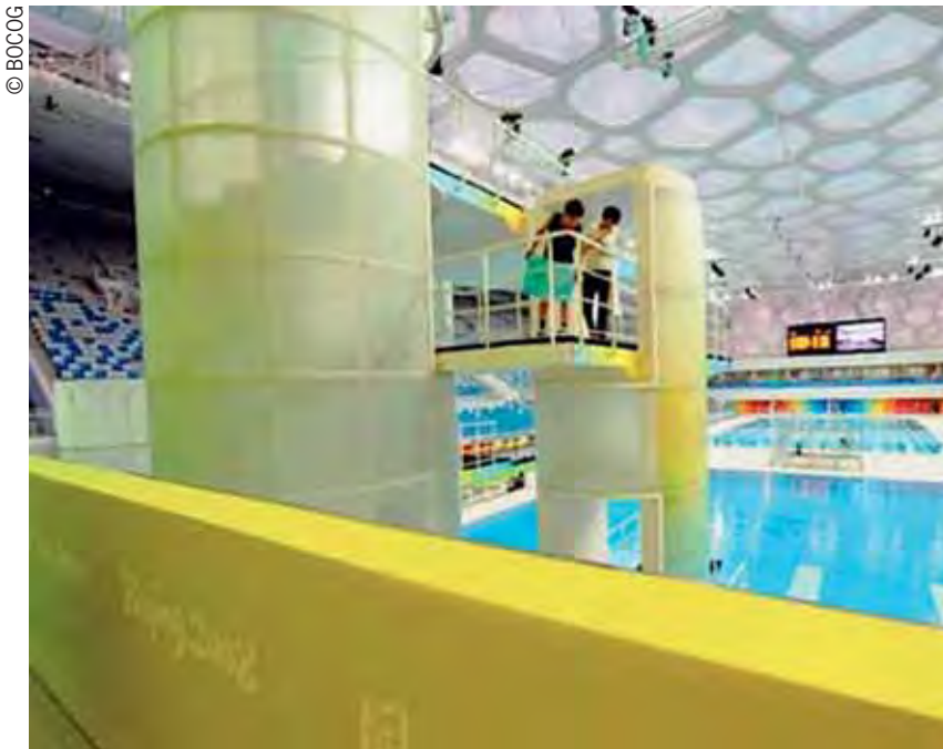
Anti-penetration concrete was among the water saving features at the Water Cube (below and right).
