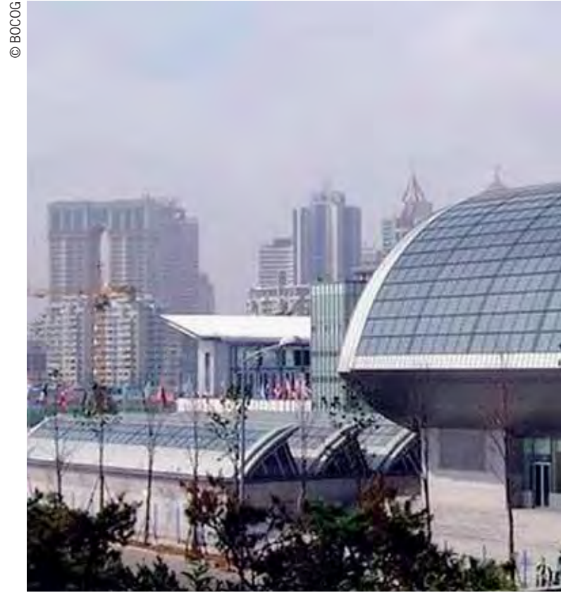
Stricter environmental building guidelines are recommended for future Games.
