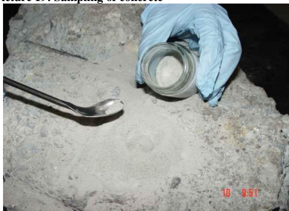
Picture 19: Sampling of concrete
