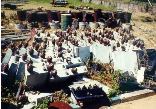
Picture 84: Bad example I (open air storage)
