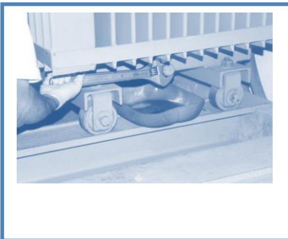
Place drip tray under drain tap, wearing gloves and goggles
