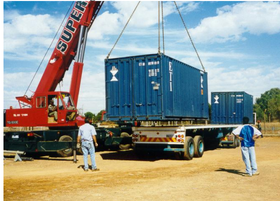
Picture 98: Lifting of containers to truck
