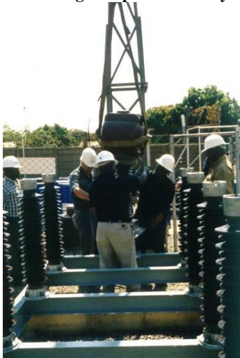
Picture 55: Dismantling of capacitor battery
