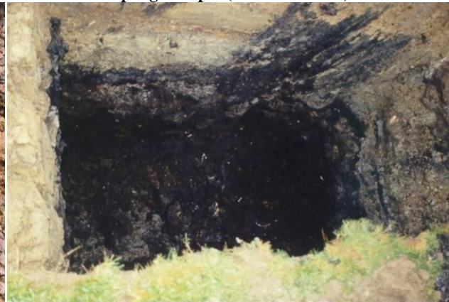
Picture 22: Sampling in depth (Excavation slot)
