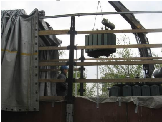
Picture 71: Loading of transformers
