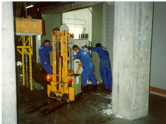
Picture 54: Phase out of an intact PCB transformer
