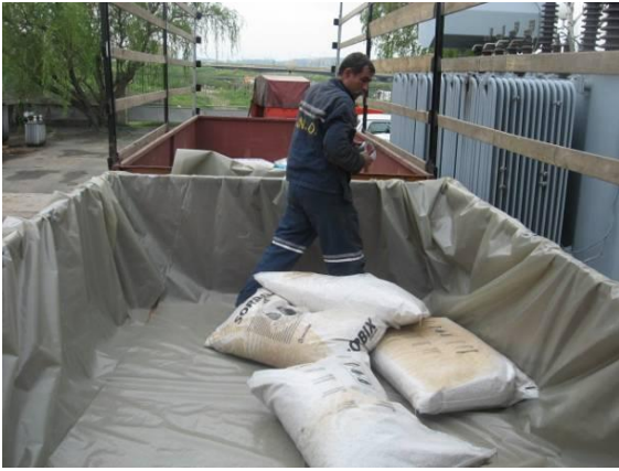
Picture 69: Preparation: transportation of PCB transformer
