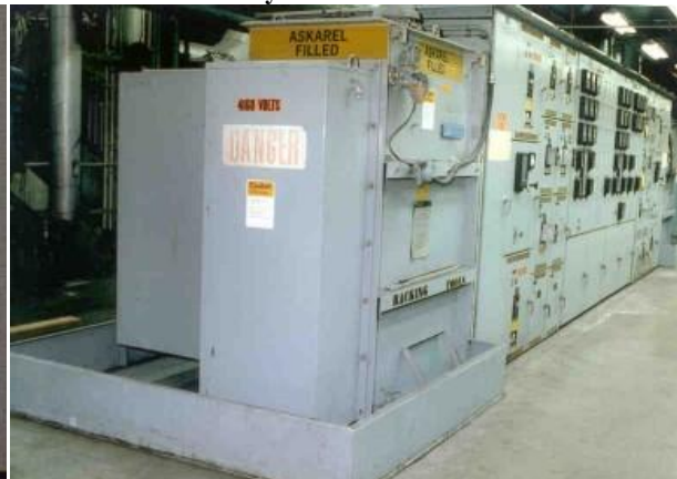
Picture 39: Retention system made from steel
