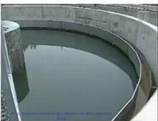
Waste water treatment plants
