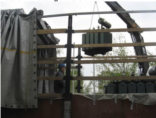
Picture 71: Loading of transformers
