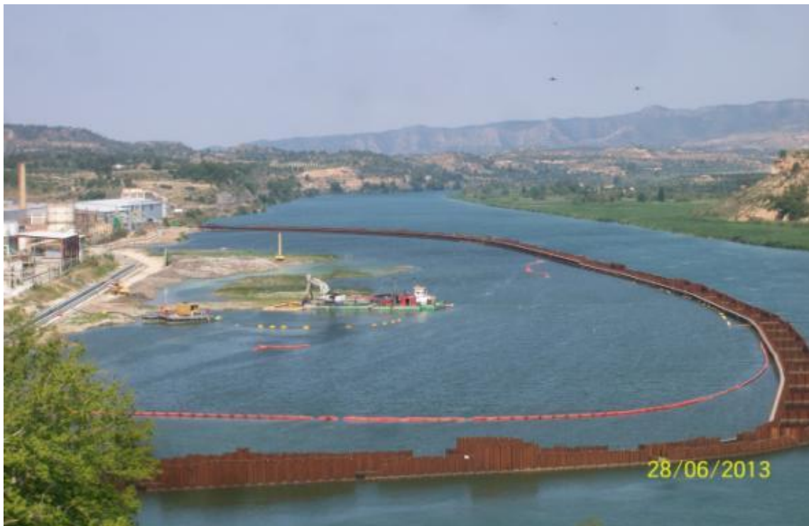
Dredging activities inside the sheet piling
