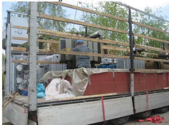
Picture 72: Stowing of transformers
