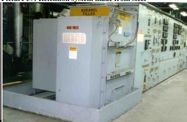
Picture 39: Retention system made from steel
