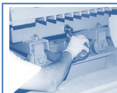
Sample the oil (30-50ml for PCB screening, 1l if also oil quality is tested)
