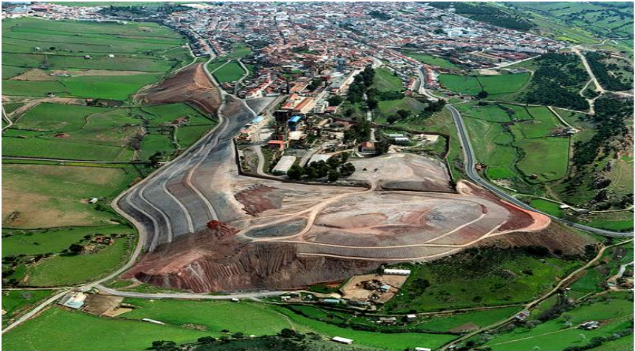
REMODELLING OF THE CERCO DE SAN TEODORO SLAG HEAP MARCH 2006. Photo by Paisajes Españoles
