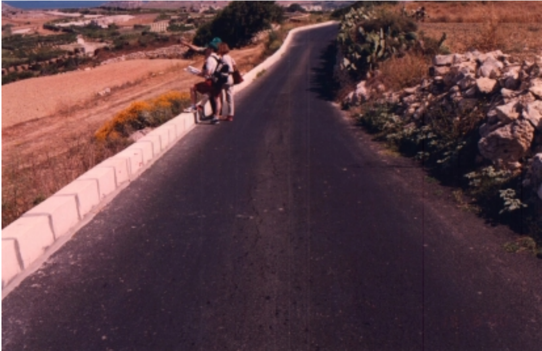
Plate VI. 23. Following the November 1999 storm, a new asphalt road was laid down with one course layer of stone blocks built along the perimeter of the road to divert storm water, Tas-Santi
