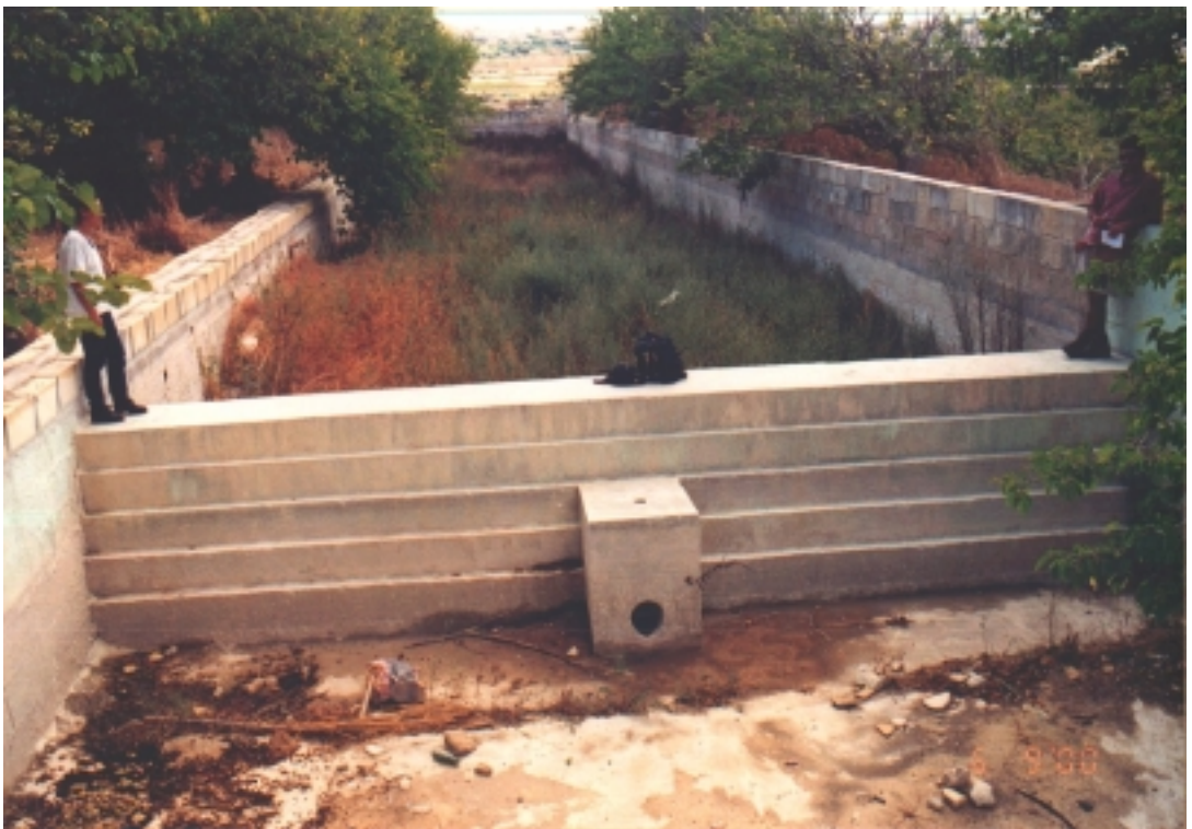
Plate V.3. Sediment trap, WSC Station, Burmarrad, 2000
