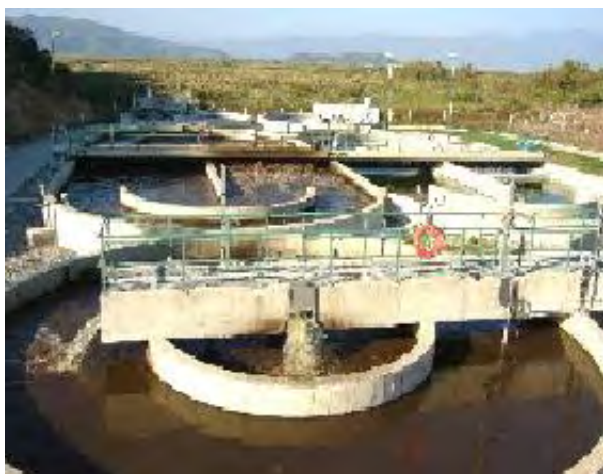
Picture 3 Dalyan Waste Water Refinery
