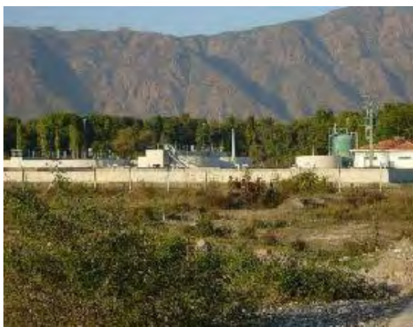
Picture 1 Köyceğiz Waste Water Refinery
