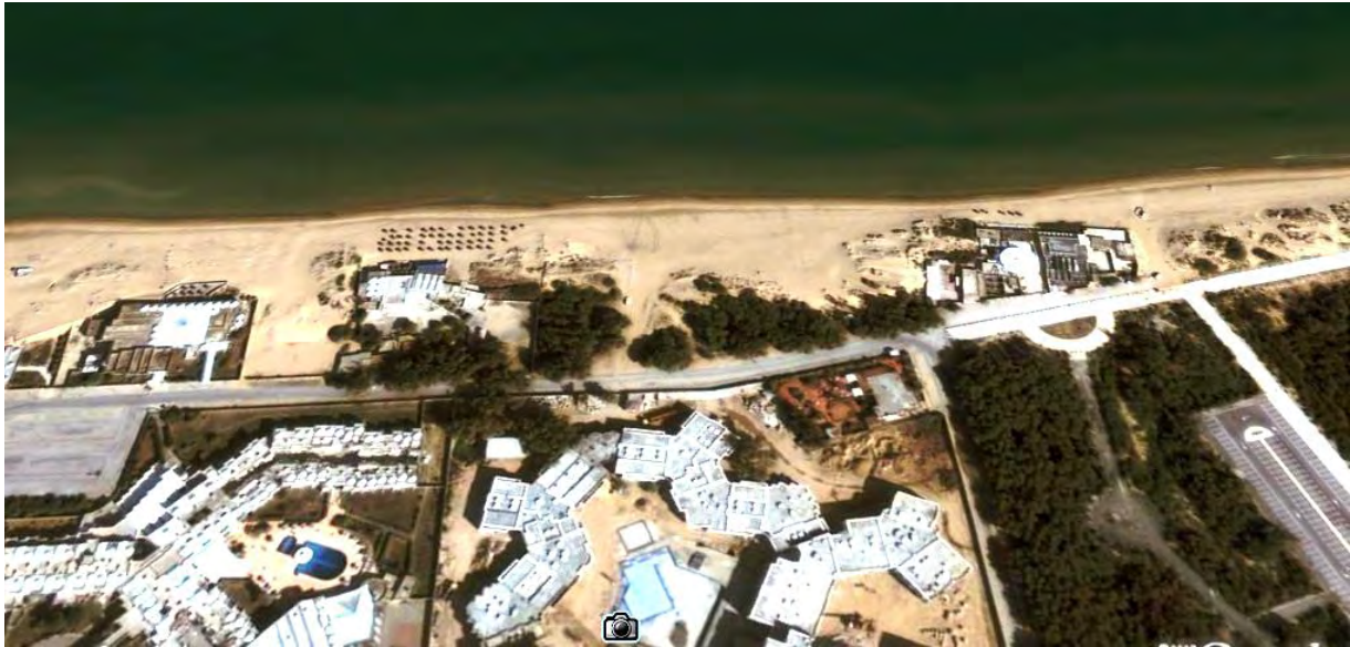
Figure 3 Construction on the dunes in the Mediterranean
