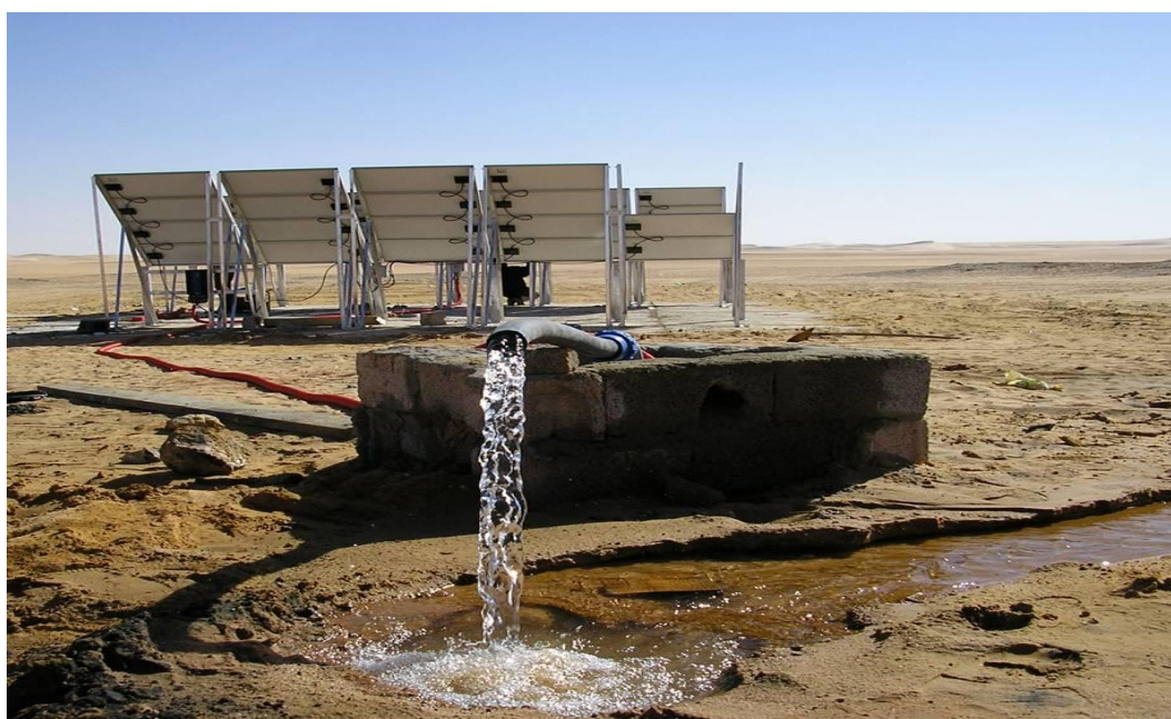
Figure 22 PV Water Pumping Beer Tssawa
