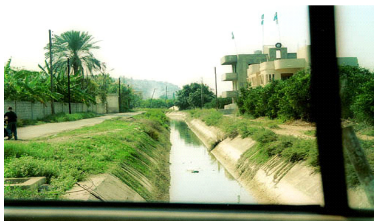
Photo 46: Irrigation channel, Sarafand (Litani project)
