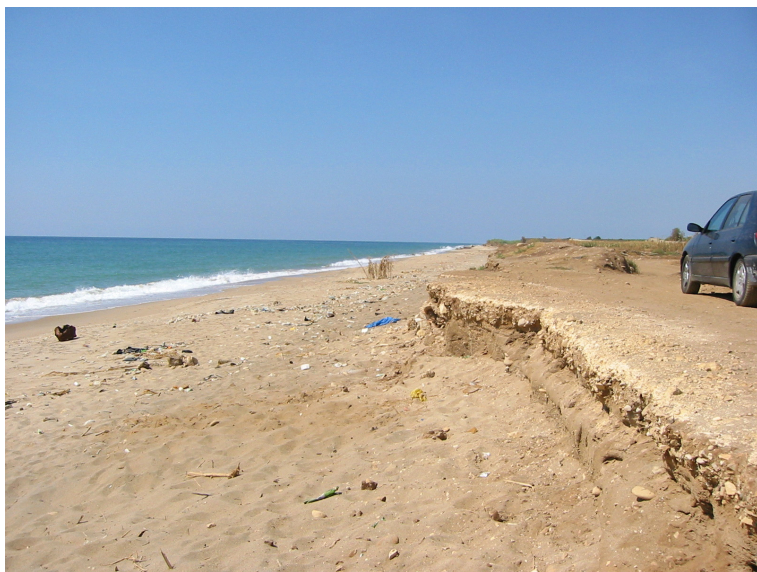
Photo 17: Beach erosion and subsidence
