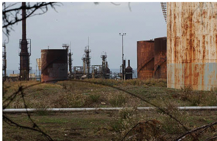
Photo 41: Decommissioned petroleum refinery in Zahrani
