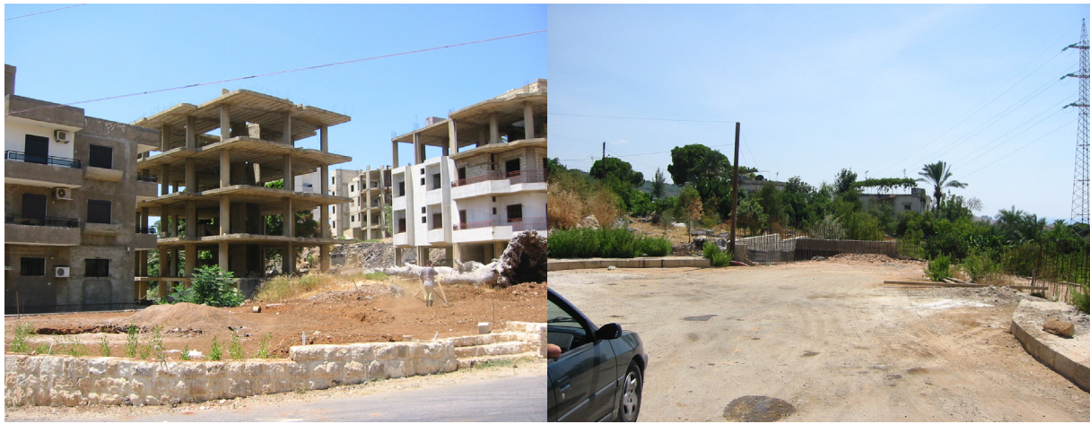
Photo 13, Photo 14: Examples of construction works
