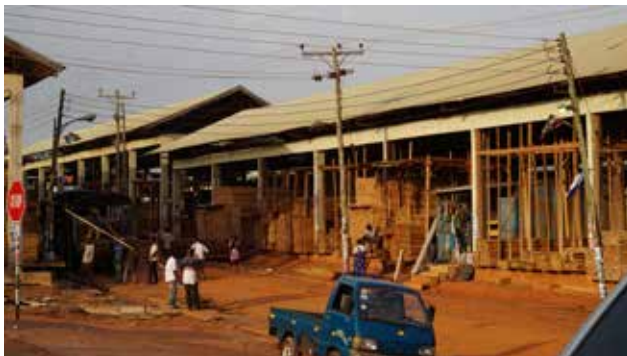
Section where timber is stored at Sokoban Wood Village, showing the busy activity at the business premises Photo | SWITCH Africa Green
