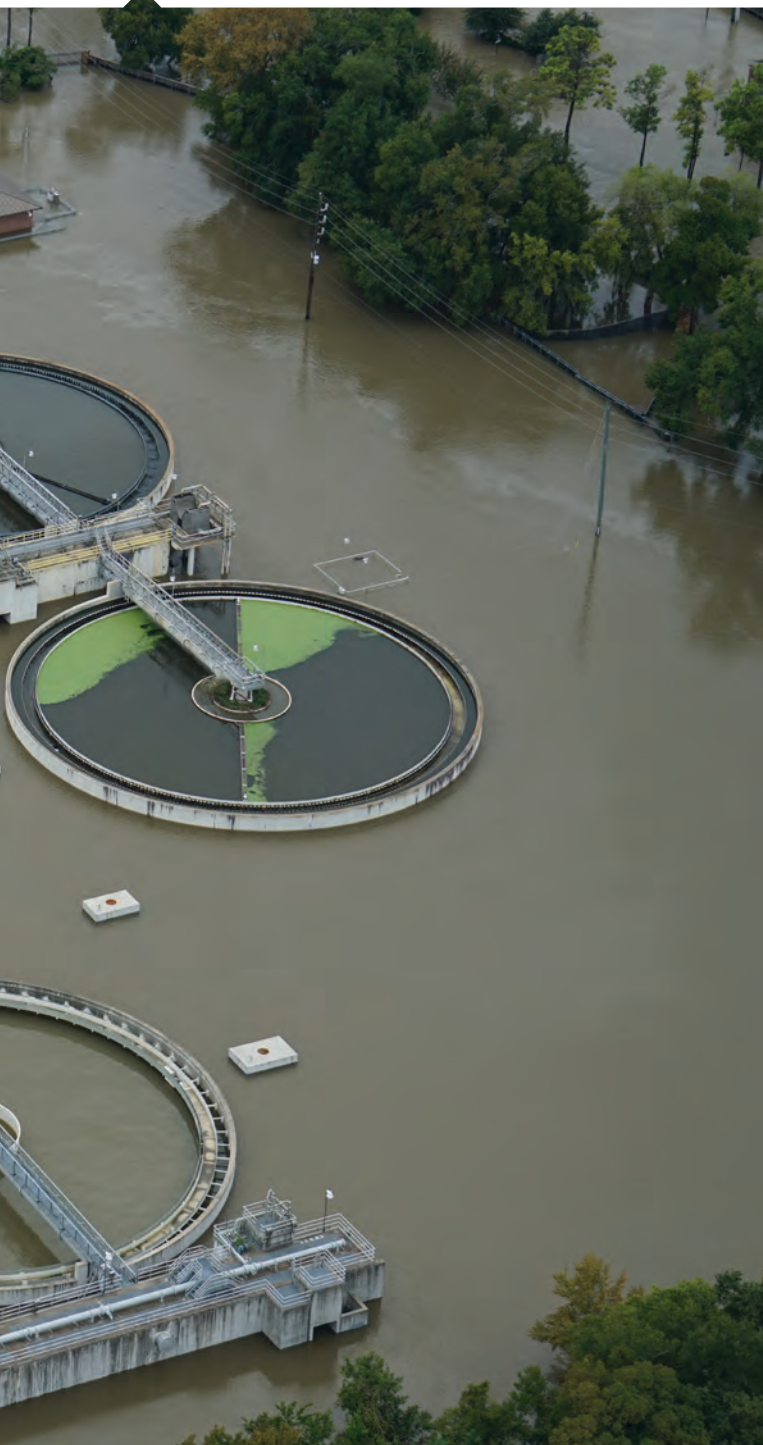
Flooded wastewater treatment plant after Hurricane Harvey (USA)
