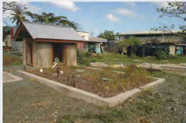
Construction of Wetland Filtration Unit
