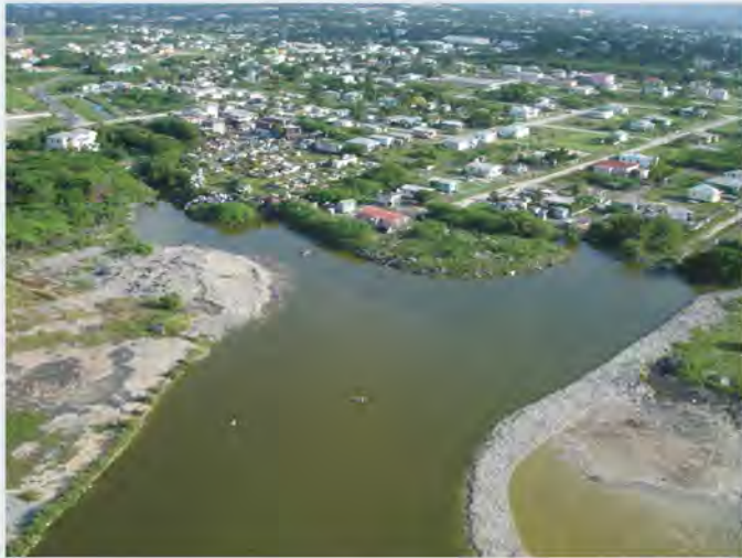
McKinnon's Pond, Antigua Demo site
