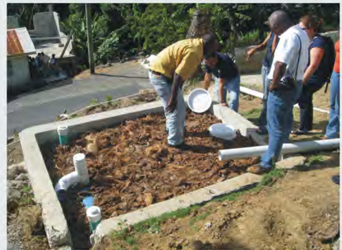
Construction of Wetland Filtration Unit
