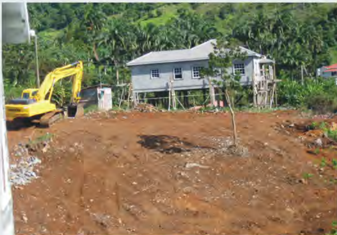
Construction and Sediment Run-Off in Grenada
