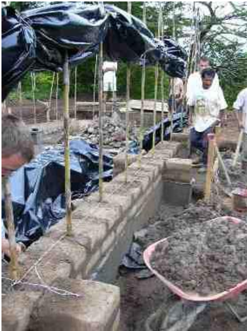
Adobe walls under construction, including plinth, pilasters, vertical and horizontal reinforcement and plastic rain-covers
