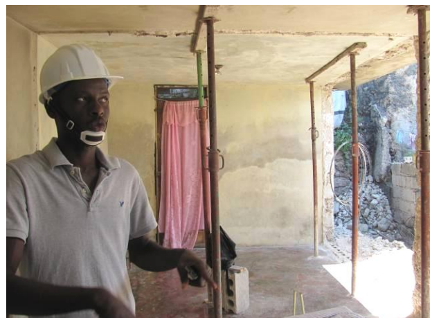
Installed props during retrofitting
