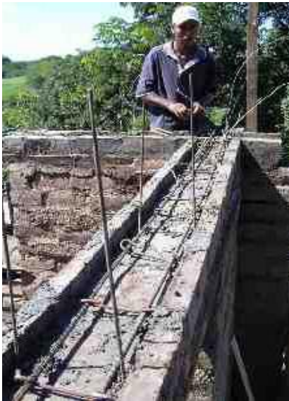
Ring beam channel blocks and reinforcement (Note: Steel pins and wire straps for roof attachment)
