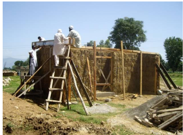
One-roomed straw-bale house under construction
