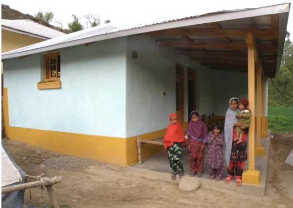
Standard 24ft x 24ft straw-bale house
