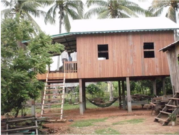
A private house on stilts
