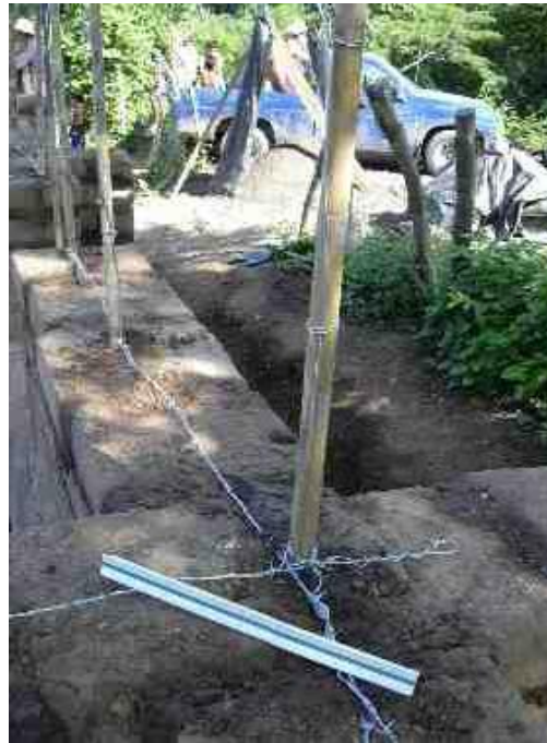
Adobe walls under construction, including plinth, pilasters, vertical and horizontal reinforcement and plastic rain-covers
