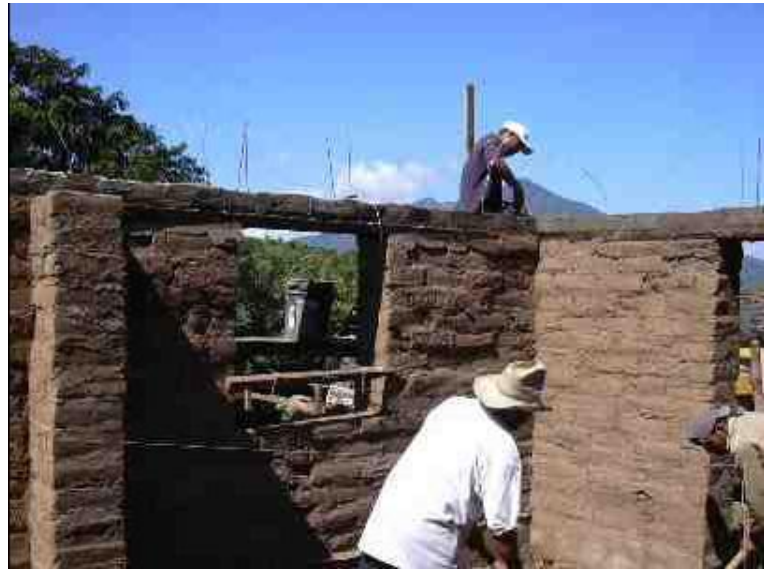
Ring beam channel blocks and reinforcement (Note: Steel pins and wire straps for roof attachment)
