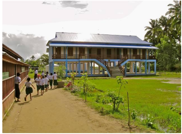
Elevating the ground floor of a school
