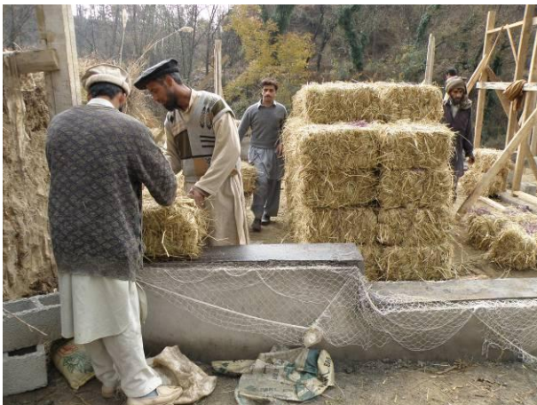
Placing first layer of straw bales
