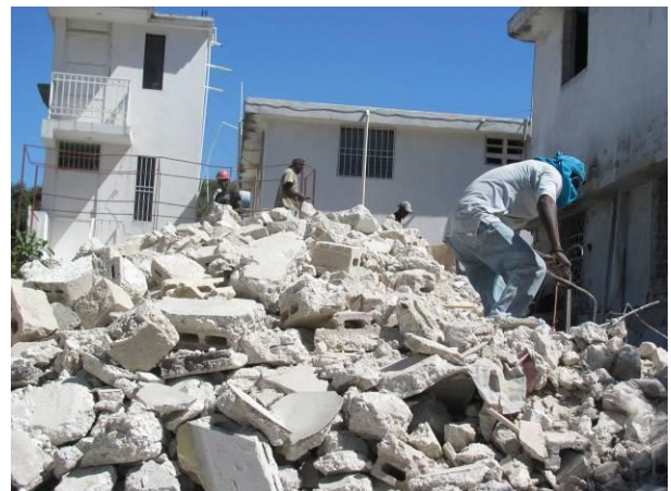
Demolition works in Haiti
