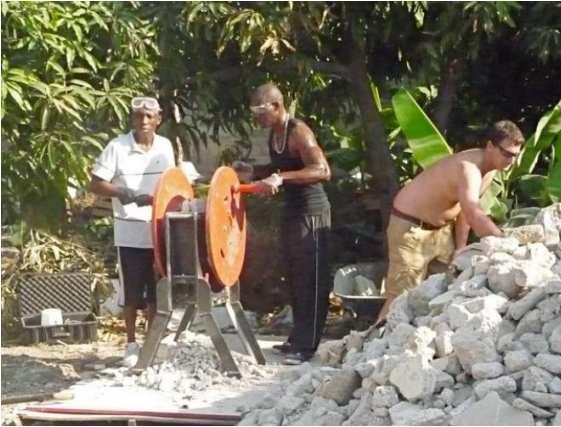
Crushing rubble into usable aggregate
