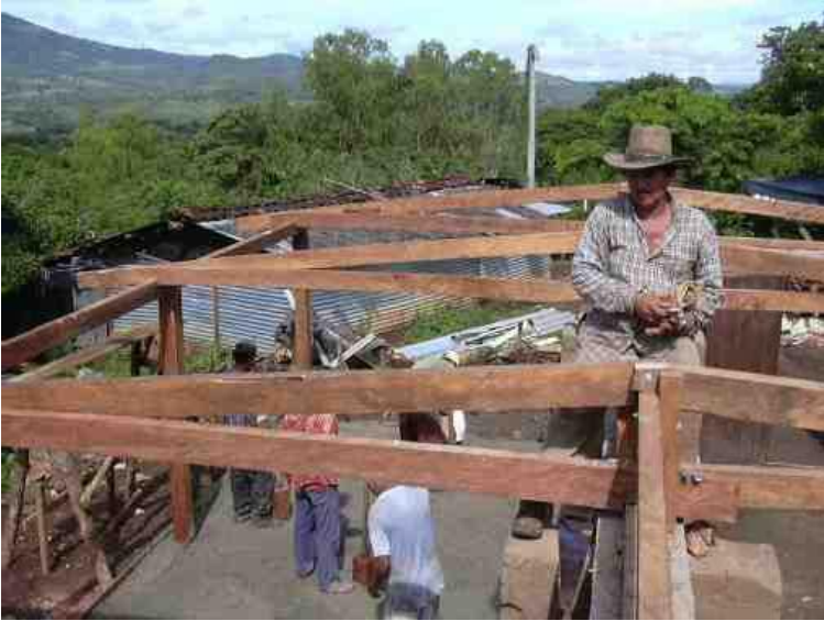
Roof under construction
