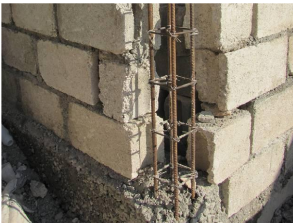
Reinforcement and connection of external walls
