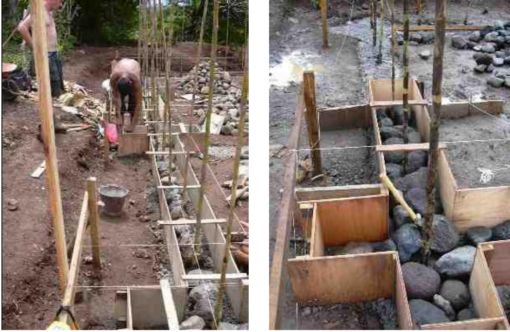
Location of vertical reinforcement and preparation of plinth formwork
