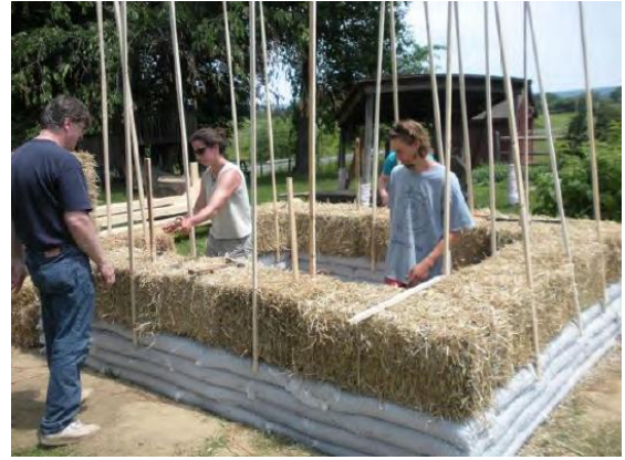
Construction of straw-bale walls
