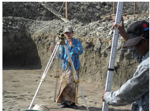
Surveyors at work
