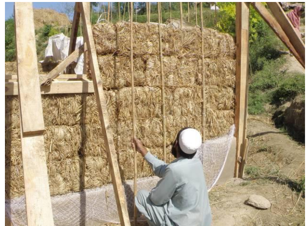
Bamboo pins provide out-of-plane support for straw-bale walls
