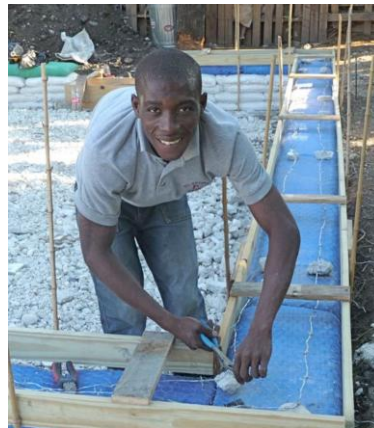
Preparations for wall construction
