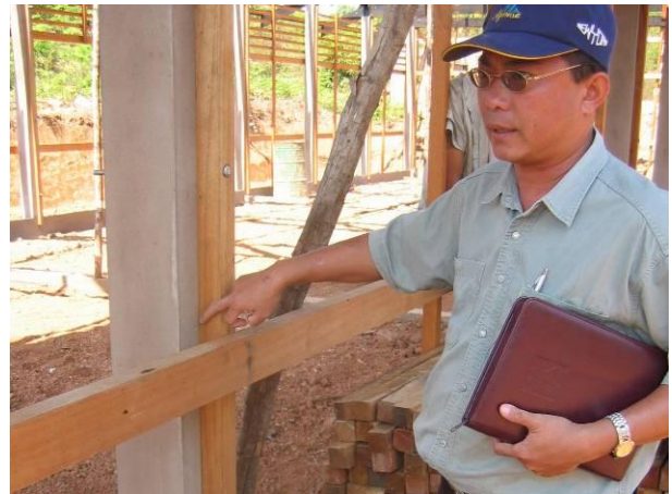
Quality check at construction site
