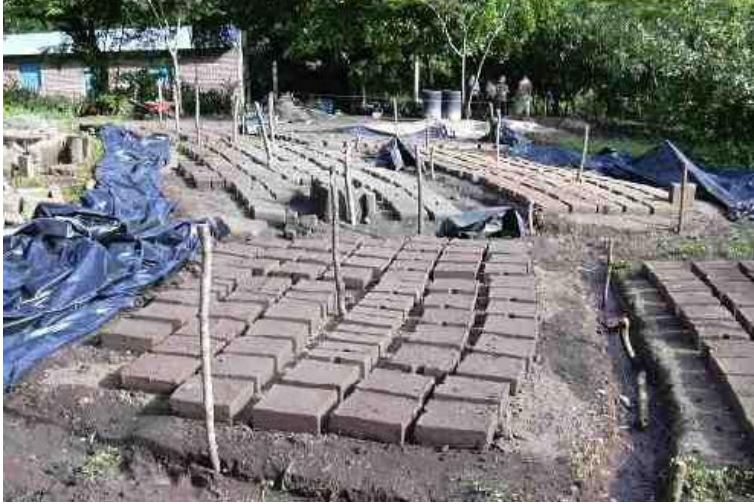
Drying bricks (Note: Drainage ditches and plastic covers)
