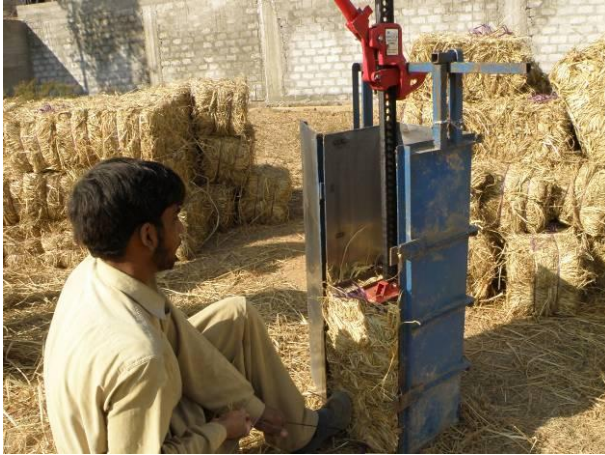
Fabricating straw bales on site
