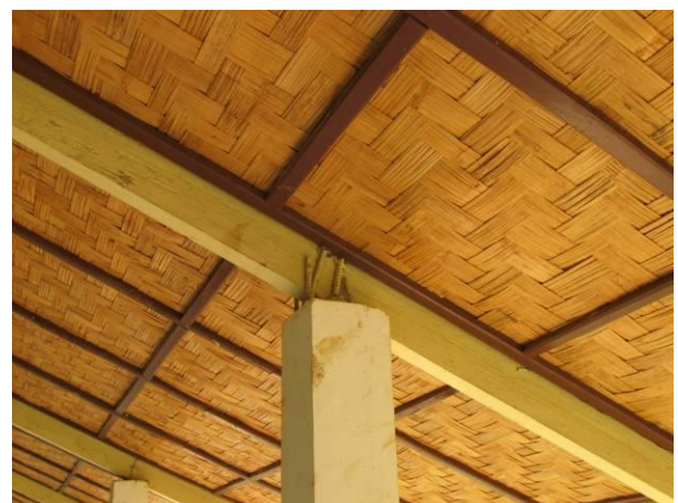
Roof is tightly connected to columns
