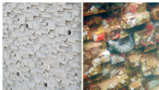
Figure 1. Eco Seawall, before installation (left); and after 12 months (right).
