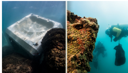
Figure 2. Eco Armor Block, minutes after installation (left); and after 24 months (right).
